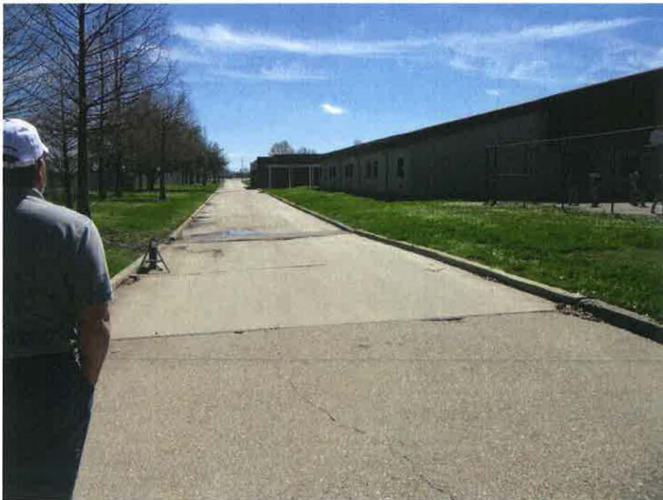
View of eastern portion of APE facing south, East St. John High School Eastern portions of basketball court, small classroom, and main building on right
