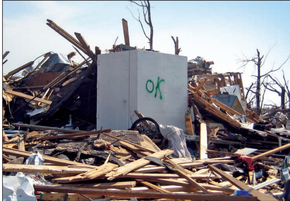
Figure 3-6: Above-ground residential safe room that was in the garage of a home hit by an EF5 tornado in Joplin, MO (2011)
