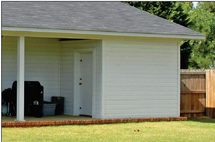
Figure 3-5: An above-ground safe room constructed as an addition to a slab-on-ground home in a way that matches the aesthetics of the house (outside Tuscaloosa, AL, 2011)
