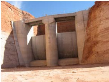
Glen Canyon Dam Gate Piers
