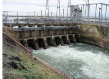
Minidoka Dam Canal Headworks Gate Piers
