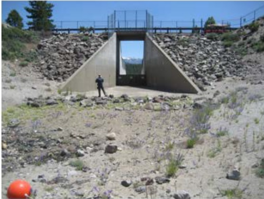
Stampede Dam Control Structure
