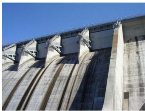
Canyon Ferry Dam Gate Piers
