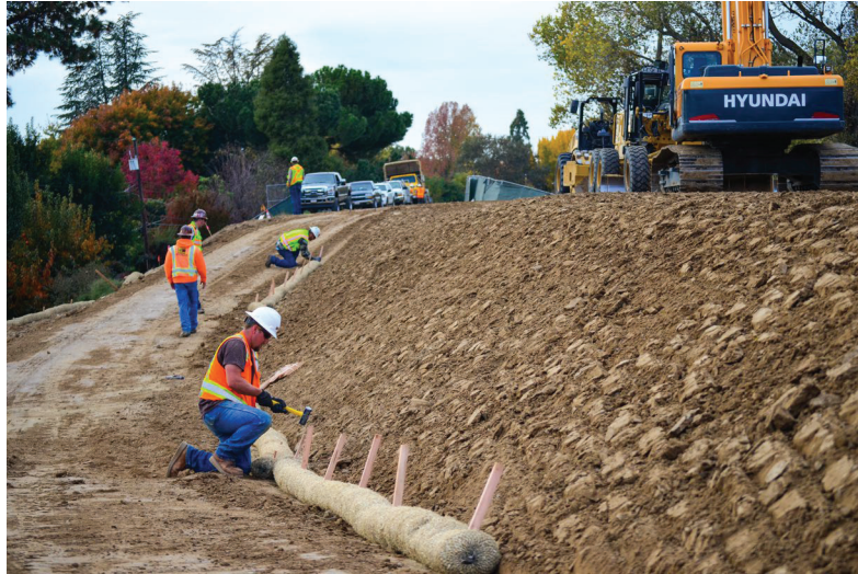
Figure 16. Fiber roll or wattle filled with straw (Todd Plain, U.S. Army Corps of Engineers, n.d.)
