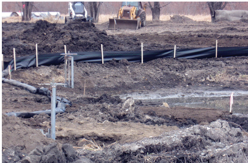
Figure 15. Silt fences and mulch can help prevent erosion after a wildfire (Gerry Shimek, USFWS, n.d.).
