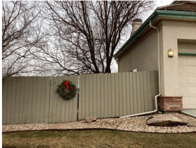
Figure 52. Combustible fencing directly attached to a single-family residence in Rock Creek Ranch in Superior, Colorado.
