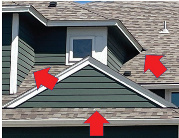
Figure 32. Example of observed areas where use of metal flashing could provide additional protections.
