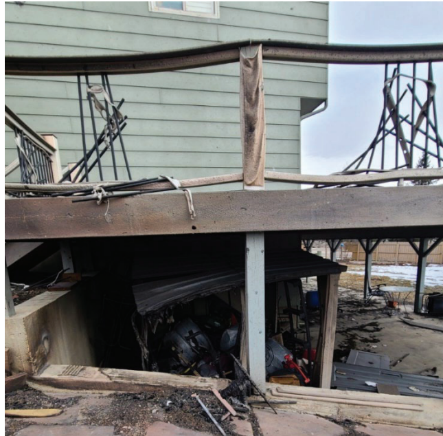
Figure 49. Elevated decks and concrete patios attached to homes were commonly observed. Many elevated decks had combustible materials stored beneath them.
