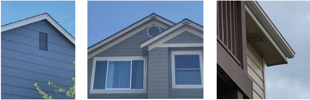
Figure 27. Lack of vent protection in attic vents, gabled roof attics, and soffits in Superior and Louisville, Colorado.
