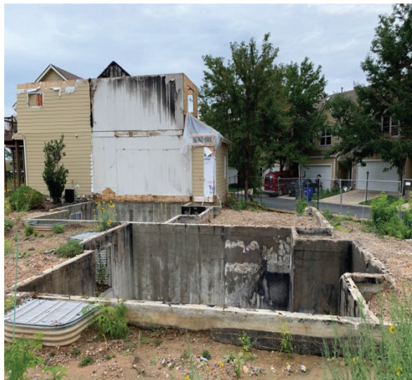
Figure 42. A Marshall Fire-damaged townhome built in 1998 in Superior with tenant separation wall not extending to underside of roof sheathing.
