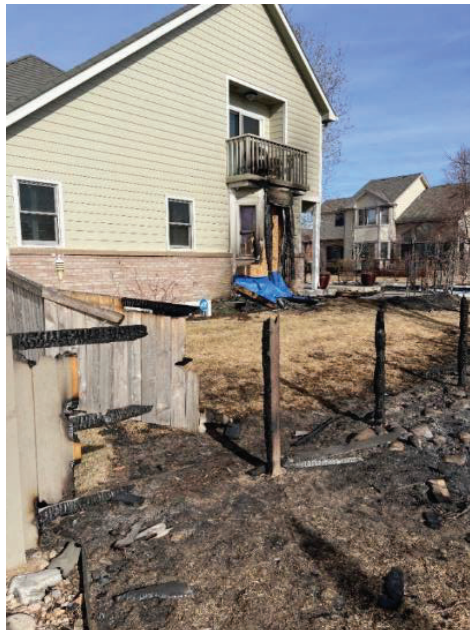
Figure 51. Balconies can catch on fire from below, which can result in spreading fire to upper levels of the house.
