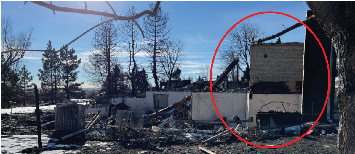
Figure 38. While blackened by smoke, soot and ash, concrete and brick elements remained standing more often than most other exterior wall construction materials.
