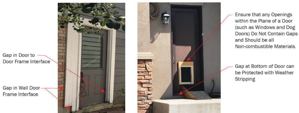
Figure 18. Examples of door-to-wall joints. Where openings in the plane of a door exist, such as dog doors or windows, the gaps around the openings should be filled caulking, mineral wool, or similar non-combustible material. In addition, the opening itself should be protected from ember intrusion that can be deployed during a wildfire incident (e.g., provide a noncombustible shutter).
