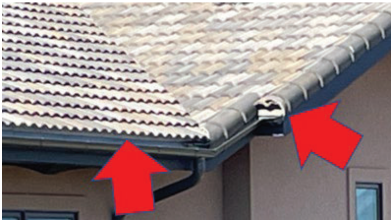
Figure 35. Example of observed profile-tiled roof with gaps at the roof edge.
