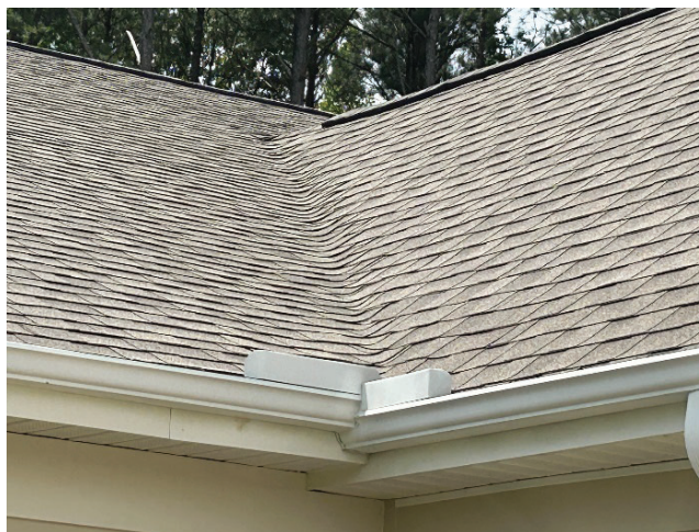
Figure 31. Example of a woven valley.
