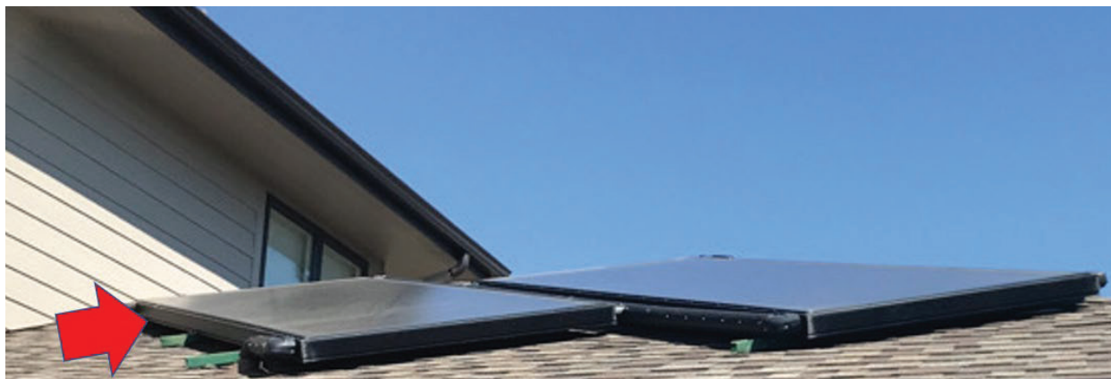
Figure 29. Example of observed unprotected solar panel installation.
