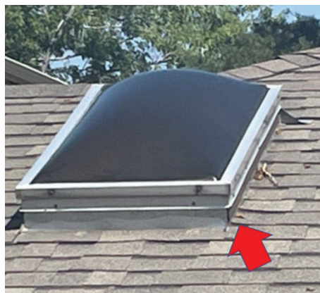
Figure 34. Example of metal flashing at joint between the skylight unit and the roof.
