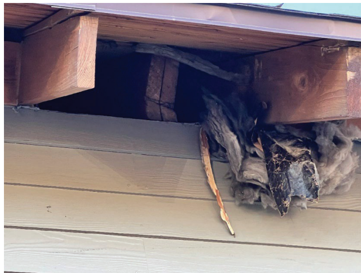
Figure 28. Wood blocking or attic vents blow out possibly due to high winds.
