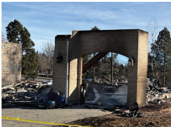
Figure 39. Concrete block and brick around garages often remained partially or fully standing.
