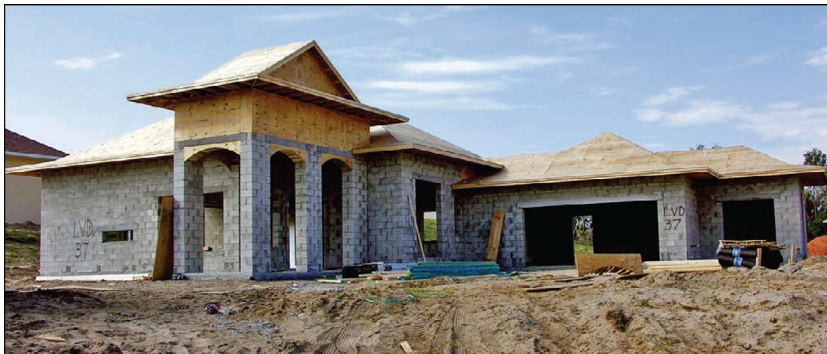
Figure 3-3: Exterior walls constructed of CMU (New Smyrna Beach, FL, 2007)
