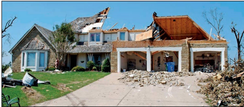
Figure 2-7: Example of a garage door failure that likely initiated progressive failure, including loss of the garage roof (Joplin, MO; EF2 rating per MAT observation)
