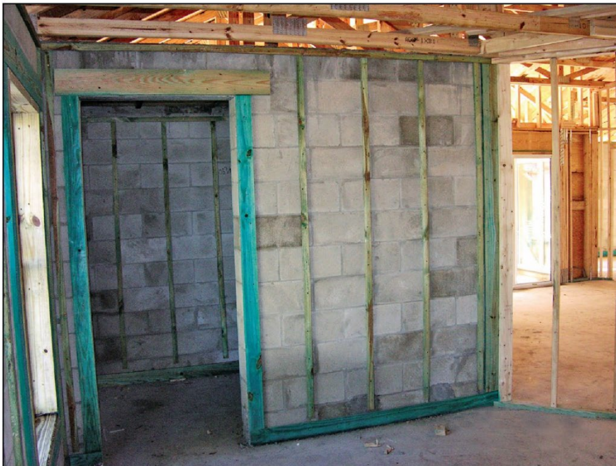
Figure 3-4: In-home safe room under construction; the CMU walls of the safe room are fully grouted and vertically reinforced with steel reinforcing bars from the foundation to the concrete roof deck (New Smyrna Beach, FL, 2007)
