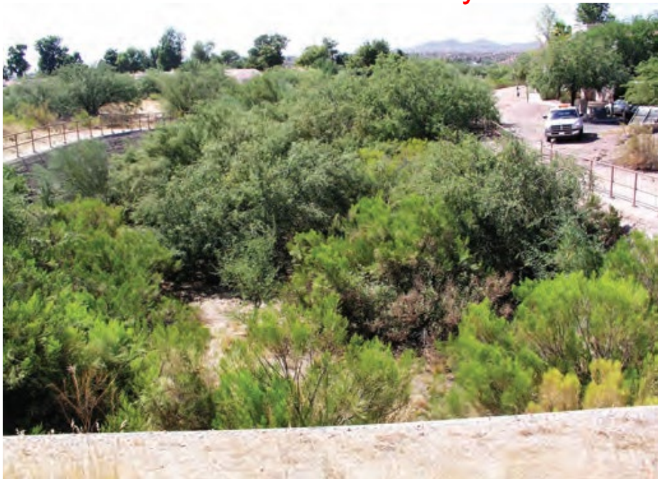
Figure 12. Picture of a constructed channel in Arizona that is overgrown with vegetation (from U.S. Geological Survey Scientific Investigations Report 2006-5108)
