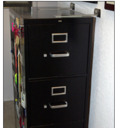
Mitigation braces hold the cabinet to wall in case of earthquake.
