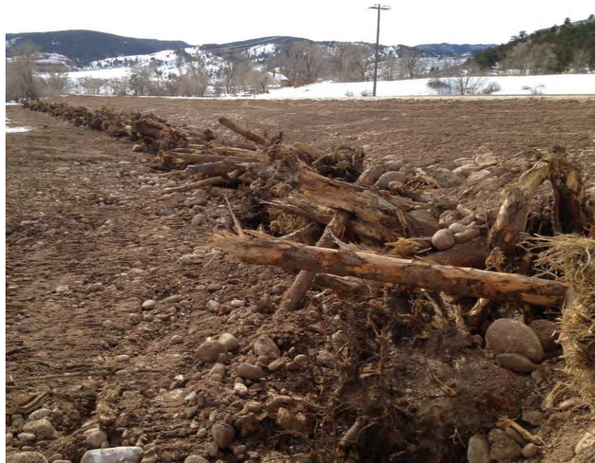
Figure 4-4: Bioengineering Using Engineered Woody Debris
