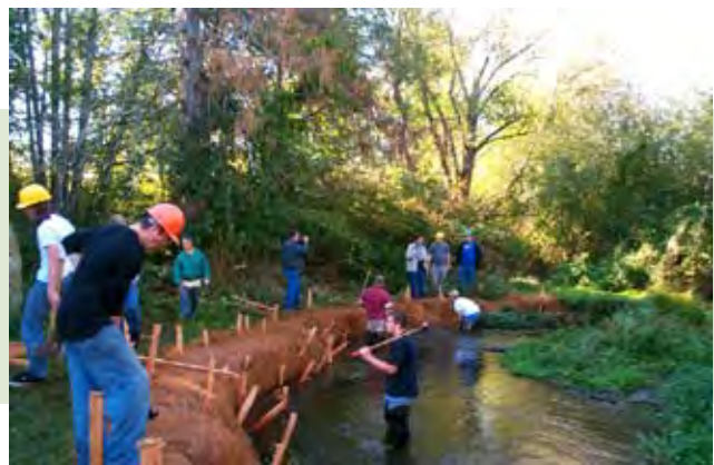
Construction of the brush mattress underway.
