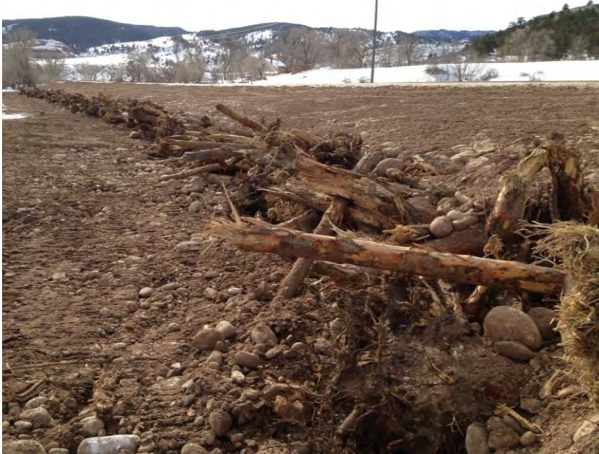
Figure 4-4: Bioengineering Using Engineered Woody Debris
