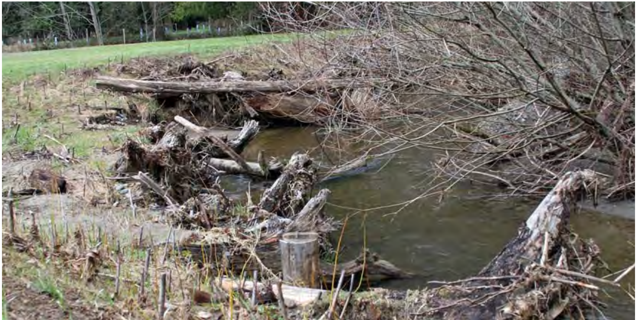
Wood added to the banks of Schneider Creek slows water flow and improves habitat diversity.
