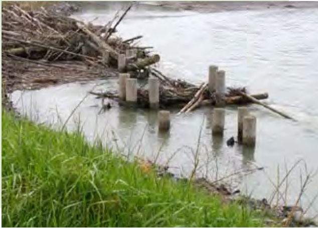
One of the scour holes being stabilized by the Overflow project. Woody debris has begun to collect and will be incorporated into the riverbank.
