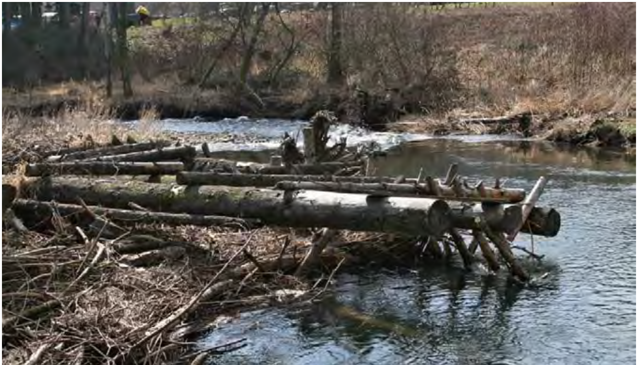
The porous design of the debris catcher allows fish to swim through the structure unimpeded.
