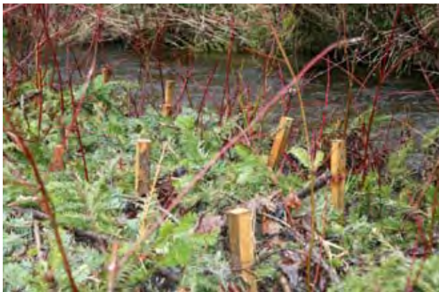
Cedar stakes driven into the creek bank provide additional soil retention.
