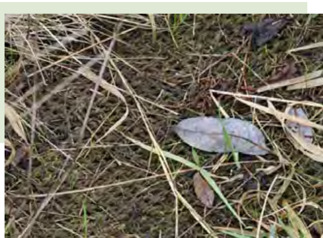
Coir fabric covers the upper bank.
