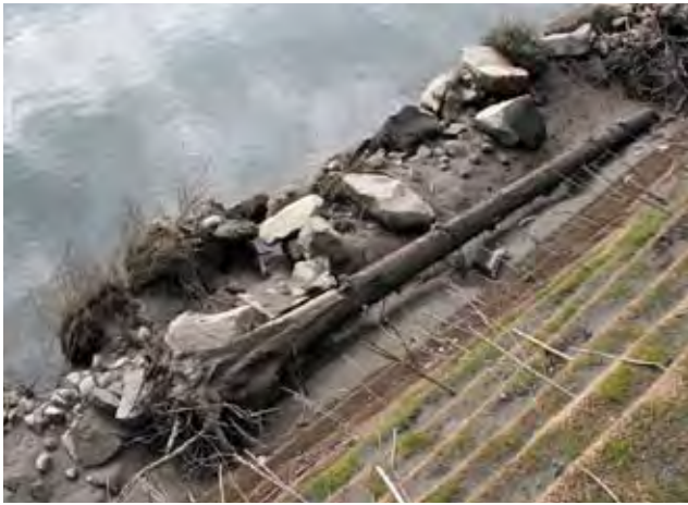
The willow cuttings planted throughout the embankment lend root cohesion and stability to the structural earth wall.
