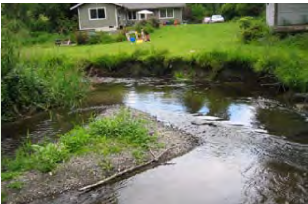
The eroding property prior to the start of the project.
