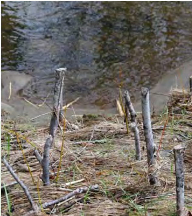
The entire bank is covered with willow cuttings for root strength.
