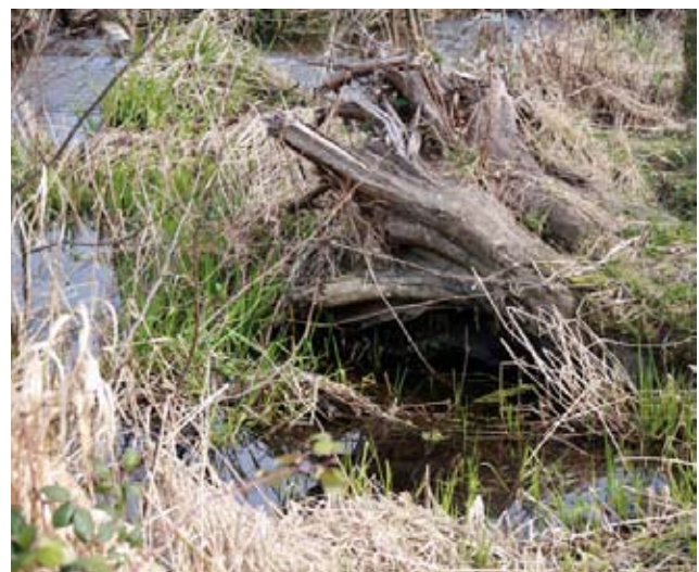
Many of the logs are actually buried in the banks.
