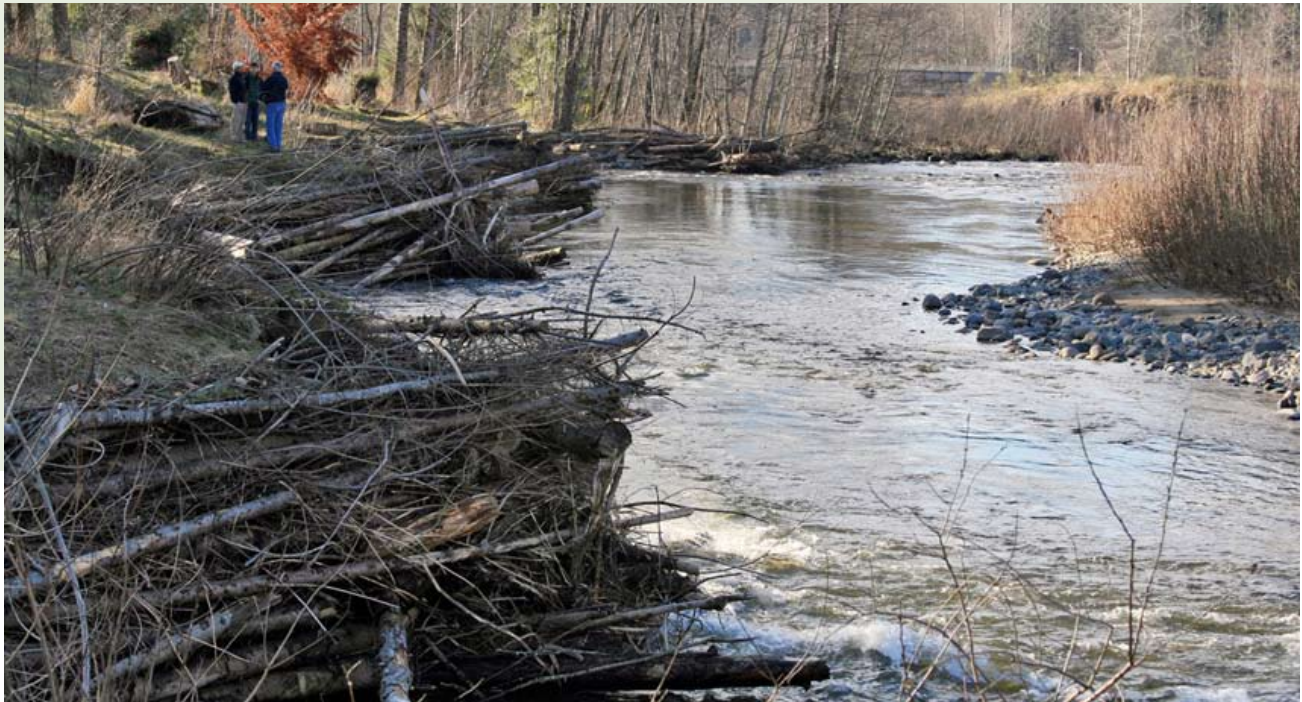
Four of the engineered logjams designed by Herrera Environmental Consultants on the Mashel River outside of Eatonville, WA.
