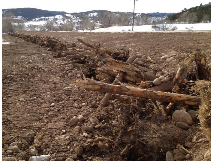
Figure 4-4: Bioengineering Using Engineered Woody Debris
