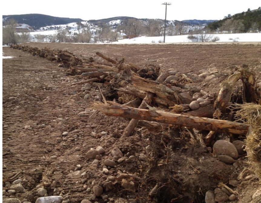
Figure 4-4: Bioengineering Using Engineered Woody Debris
