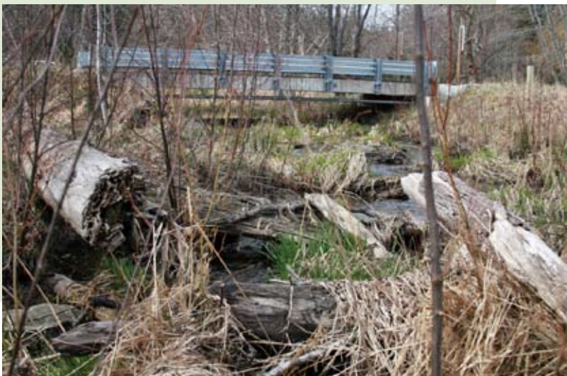
Wood positioned downstream of the bridge slows water flow and provides habitat for fish and other wildlife.
