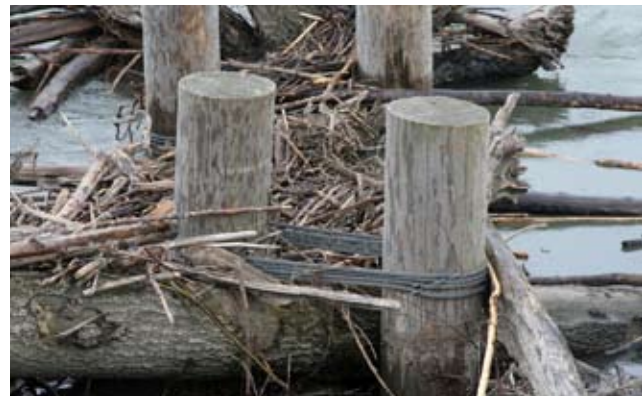
The timber piling structures capture woody debris, which provides roughness to the river, and ultimately establishes additional habitat.
