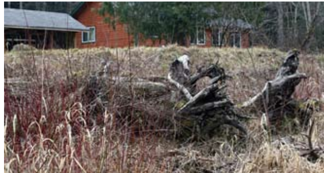
Downed trees claimed by the Forest Service provide the skeleton for the rock groin structure.
