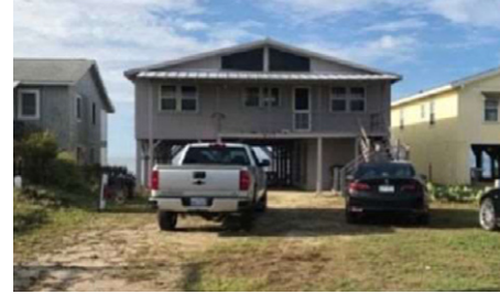
▲ Example of a sub-par photograph: photo at a distance, building obscured.
