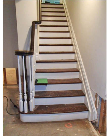
▲ Finished stairs are not covered.
