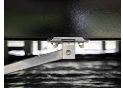
▲ Example of a tie down.
