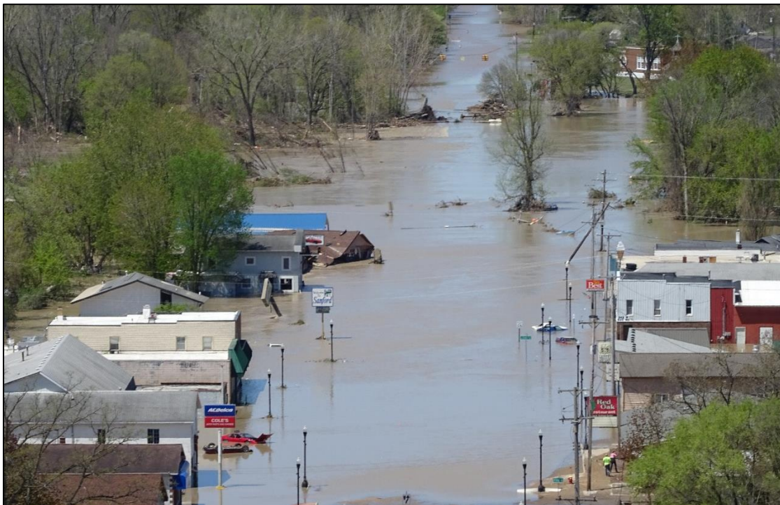
Figure 28: Downtown Sanford, just south of the Sanford Dam, after the dam failures (MSP 2022)
