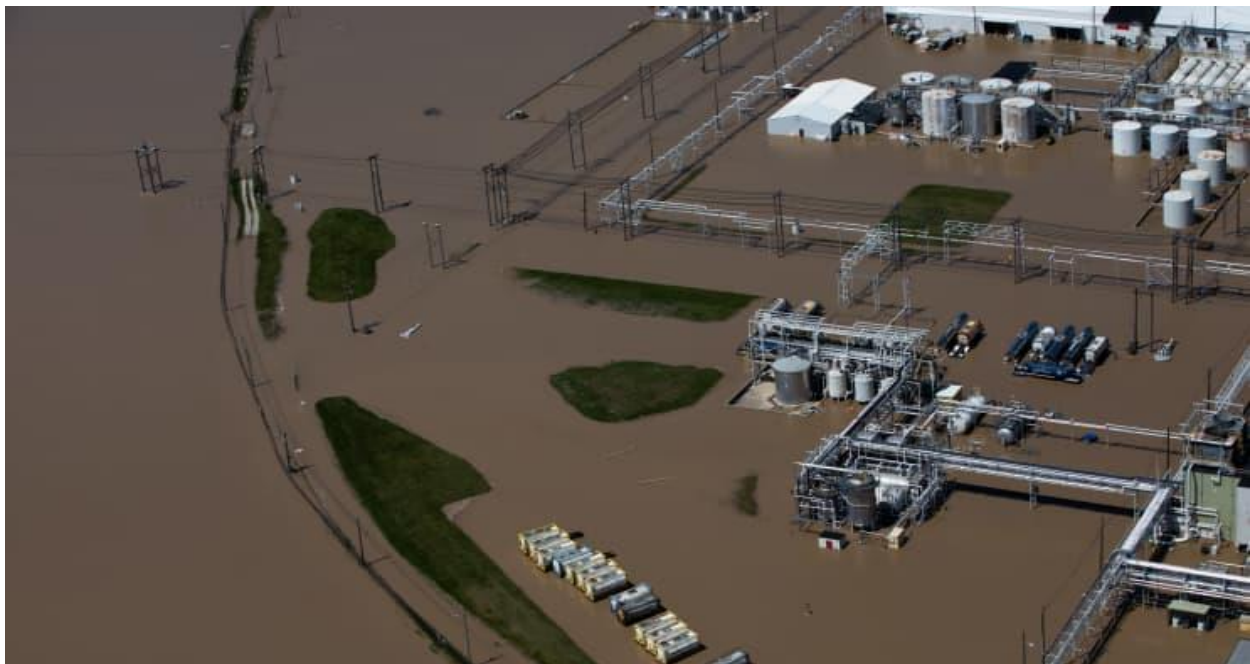
Figure 22: Dow Chemical facility along the Tittabawassee River on May 20, 2020 (Jeffery and Miller/Elconin 2020)
