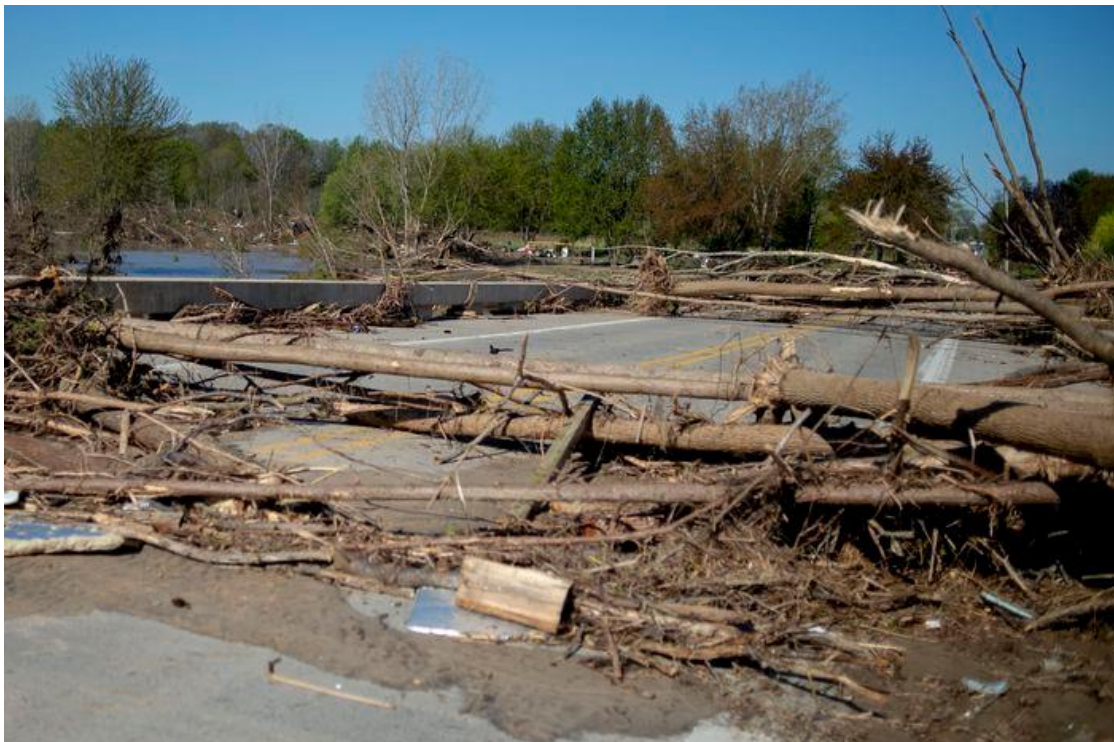
Figure 35: Debris and sediment left on Curtis Road Bridge after floodwaters receded (May 2020) (Johnson/May 2020)
