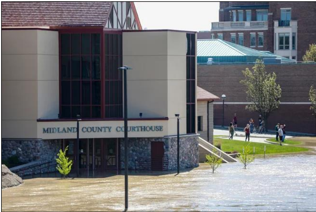
Figure 26: Midland County Courthouse in downtown Midland following the May 2020 dam failure and flooding incidents (Witsil 2020)
