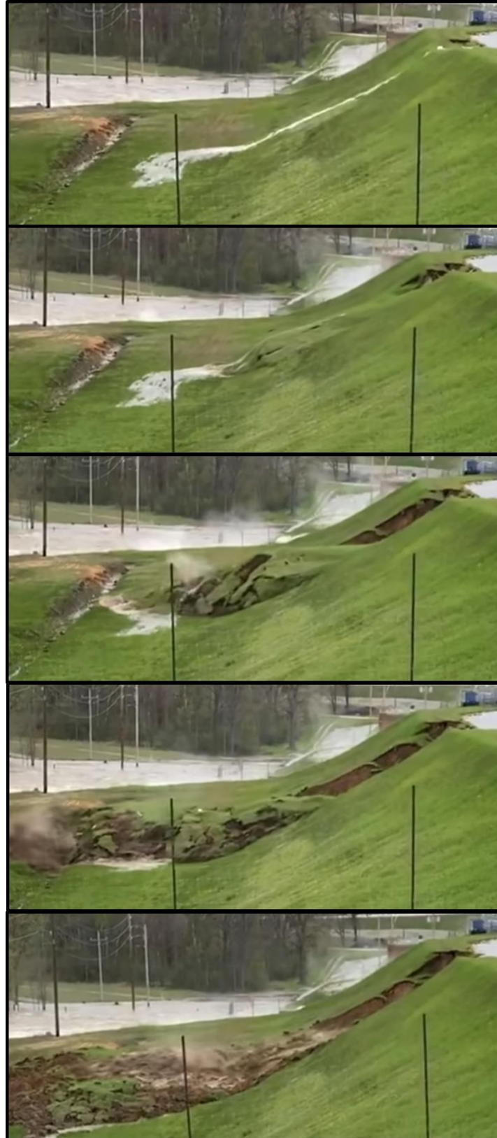
Figure 8: Progression of Edenville Dam breach along the Tittabawassee River embankment as it began, 20-second time-lapse (from top to bottom) (Coleman 2020)
