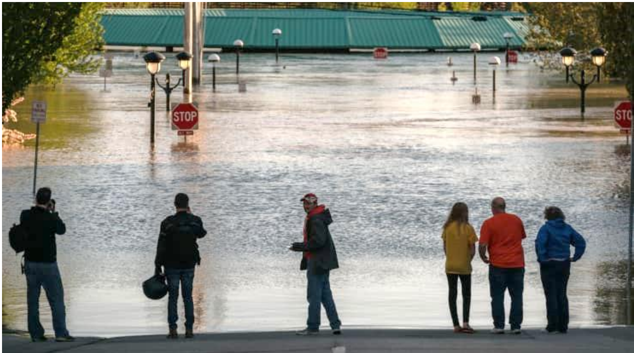
Figure 31: Midland Area Farmers Market circular pavilion following May 2020 dam failure and flooding incidents (Jeffery and Miller/Proctor 2020)
