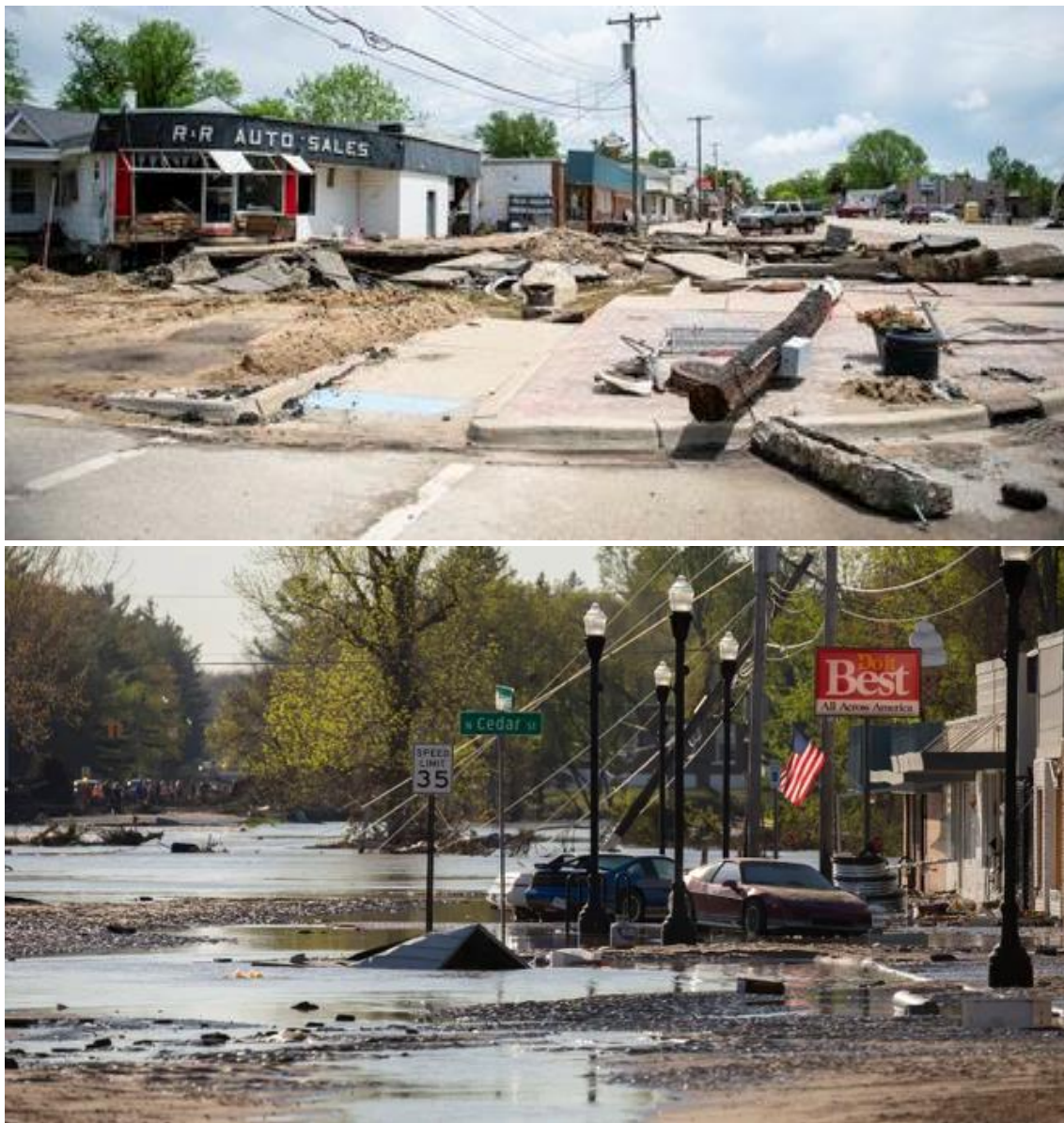
Figure 33: Debris and destruction littered the streets in downtown Sanford after floodwaters receded (Boomer 2020, Witsil 2020)
