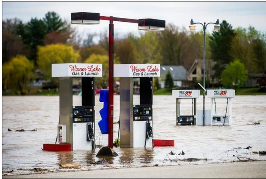
Figure 27: Flooded Wixom Lake Gas & Launch located along the west bank of the Tittabawassee River (Witsil 2020)
