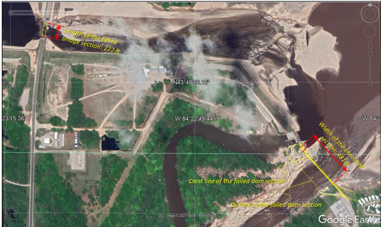
Figure 18: Aerial imagery of Edenville Dam after floodwaters receded (May 25, 2020) (Google Earth 2021)
