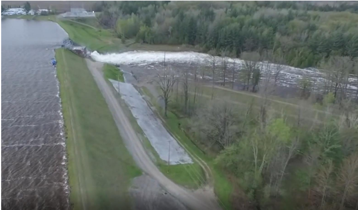
Figure 7: Tittabawassee River side embankments near capacity and fully open spillway gates on May 19, before the dam's failure (PBS 2020)
