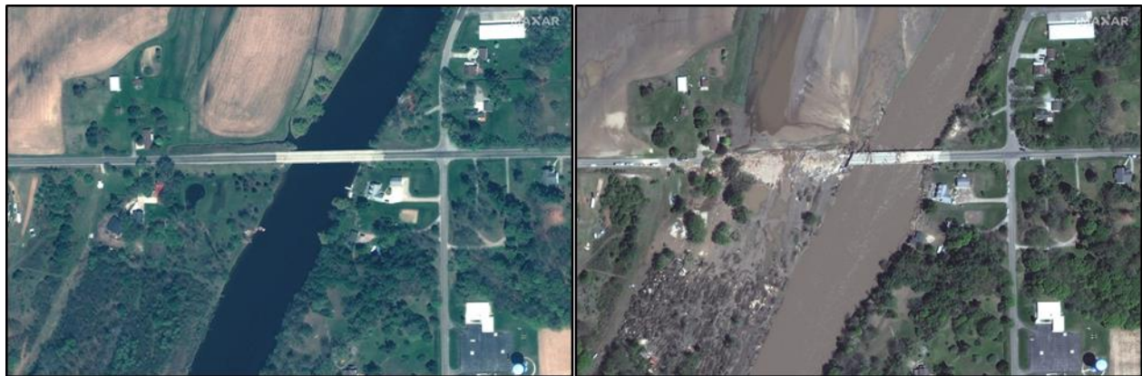
Figure 10: Curtis Road Bridge: Aerial imagery before and after the Edenville dam failure (left, May 2019, and right, May 21, 2020) (Wilkinson/Maxor 2020)
