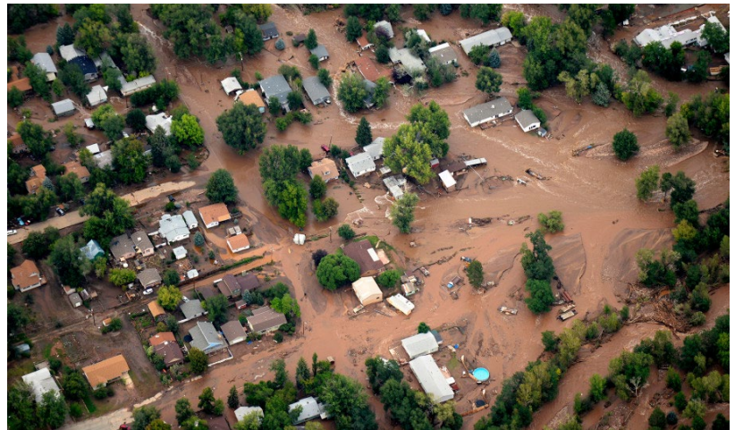
Figure 1. The town of Lyons was flooded by the North and South Vrain Creeks on September 13, 2013. Source: The Denver Post .
