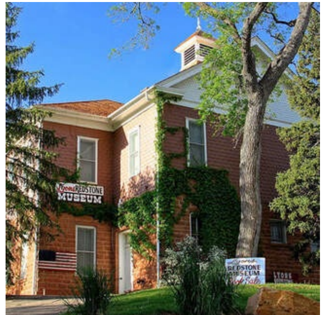
Figure 1. The Lyons Redstone Museum was damaged in the 2013 floods, but was later restored. Originally the schoolhouse in Lyons, the museum now preserves the town’s heritage through exhibits, photographs, and genealogy records. Source: Lyonscolorado.com
