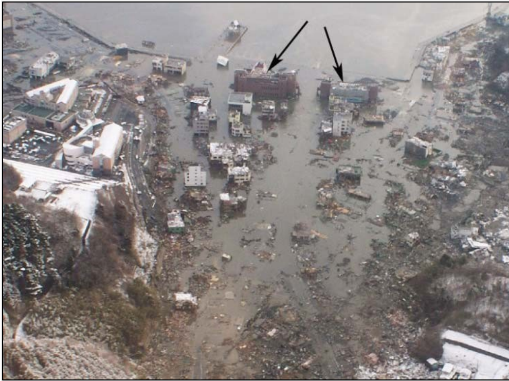
Figure 4-1 Tsunami Destruction Pattern in Onagawa, Japan 2011 Tohoku Tsunami
