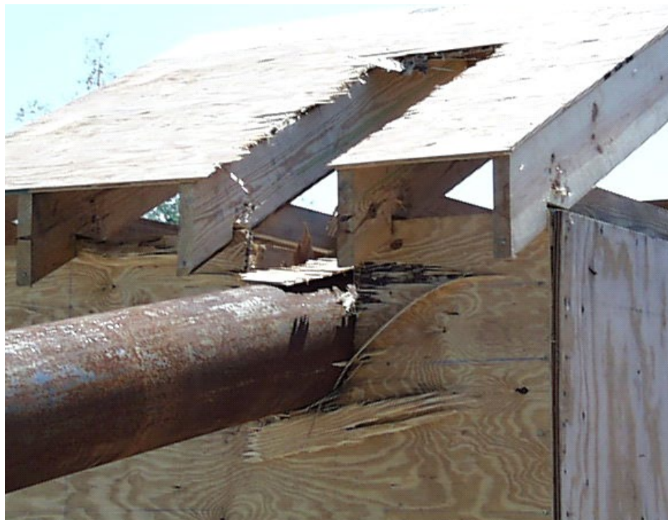
Figure 5-72 Large Pipe Impacting Roof and Wall With Plywood Sheathing, 7,600 foot-pound at Impact, Breaking Roof, Top Plates and 1/8 Wall
