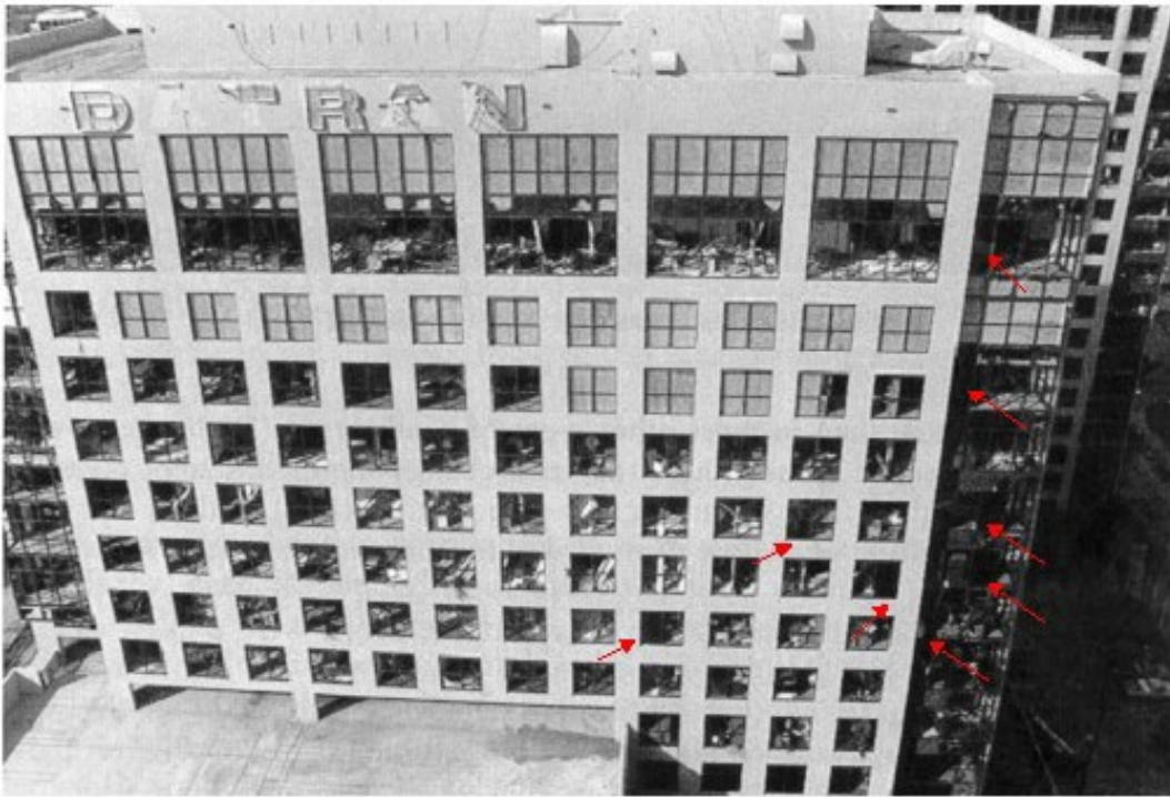
Datran Tower I, Plywood Boarding of Broken Windows Underway (Picture from Minor, 1994). Arrows indicate windows that were not damaged
