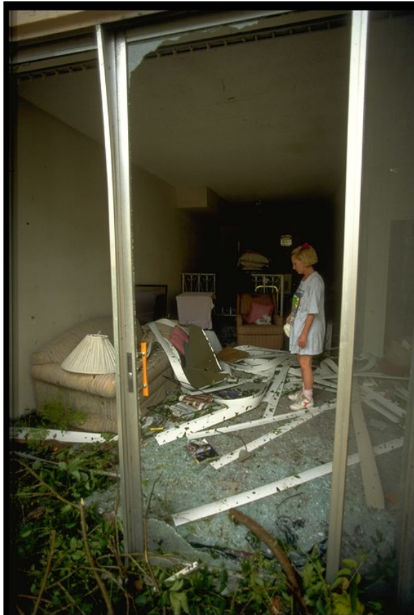
Figure 8-4 Content Losses Due to Fenestration Breach
