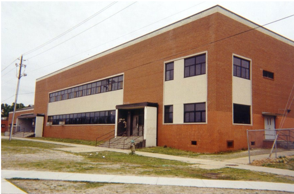
Figure 5-55 The Windward Face of the Main Missile Source Building (facing southwest)
