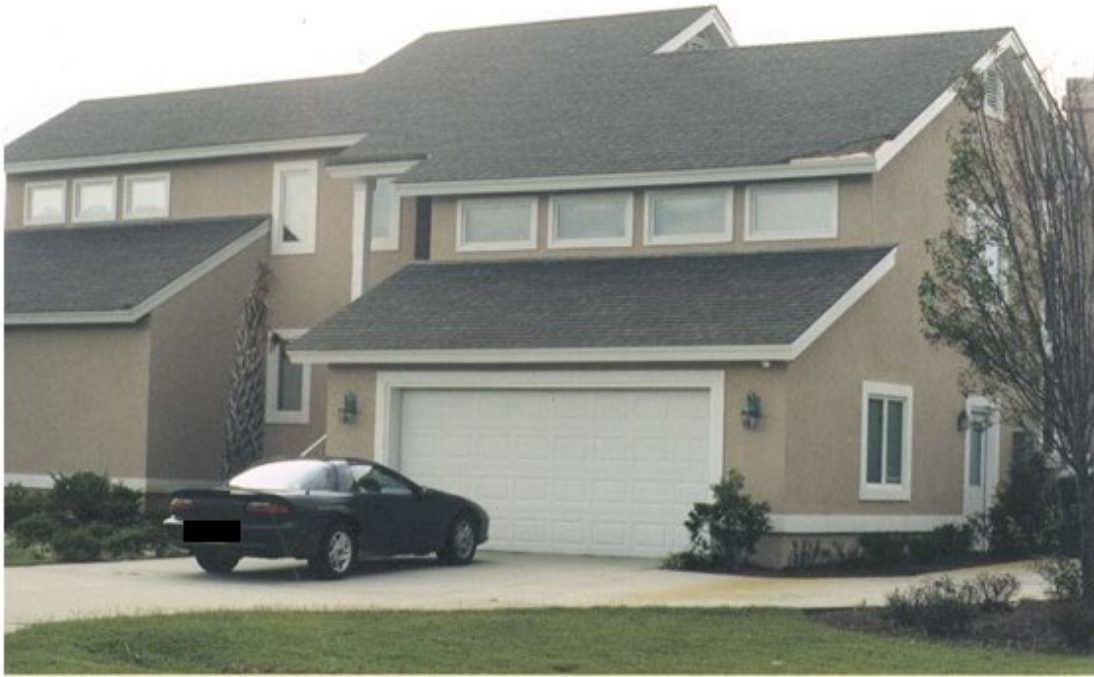
A) <2% Roof Cover
