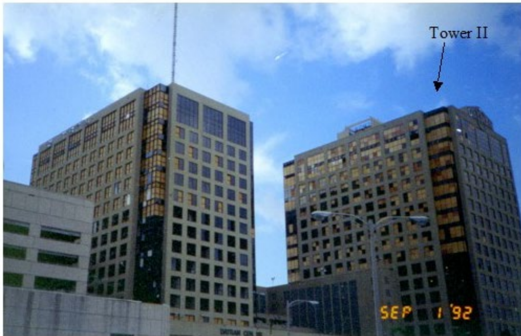
Datran Towers I and II, Plywood Boarding of Broken Windows Complete Except for Lower Floors (Courtesy of TlSmith Consulting).
