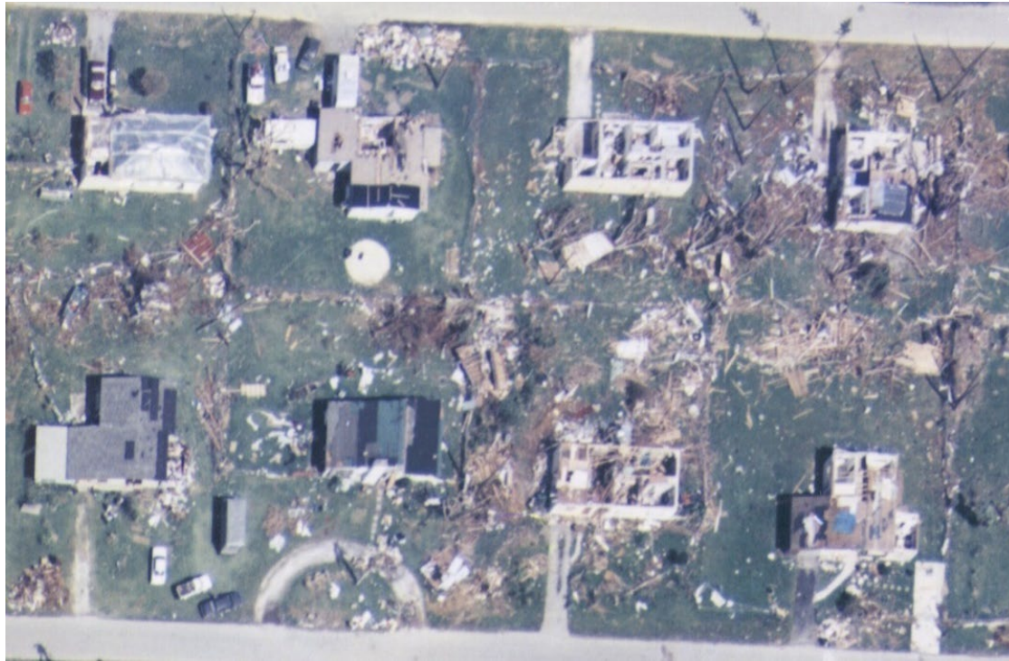
Figure 5-123 Examples of Whole Roof Failures Depicted in Photograph Number 3
