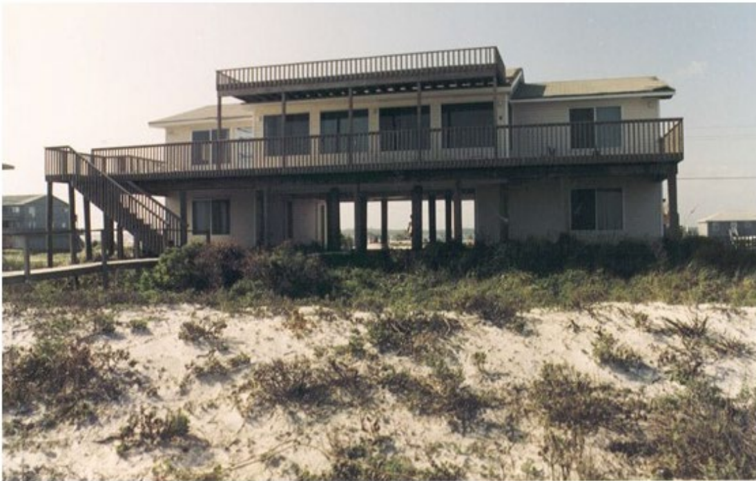
B) <2% Roof Cover
