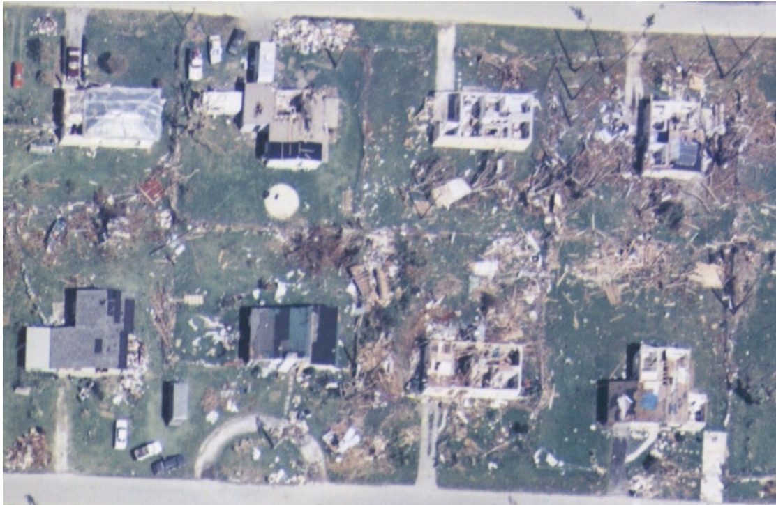
Figure 5-123 Examples of Whole Roof Failures Depicted in Photograph Number 3
