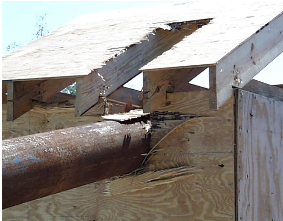
Figure 5-72 Large Pipe Impacting Roof and Wall With Plywood Sheathing, 7,600 foot-pounds at Impact, Breaking Roof, Top Plates and 1/8 Wall
