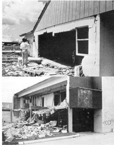
B) Collapse of masonry walls (Zollo, 1993): (top); A wall of 40' span Walls on a two-story building (bottom)
