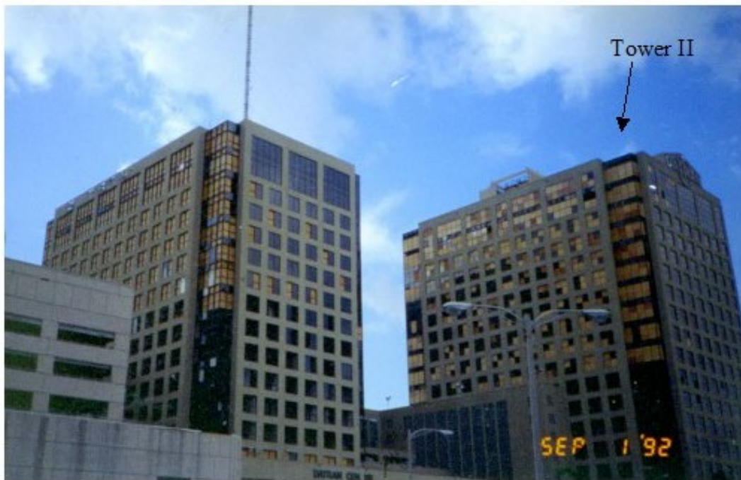
Datran Towers I and II, Plywood Boarding of Broken Windows Complete Except for Lower Floors (Courtesy of TlSmith Consulting).
