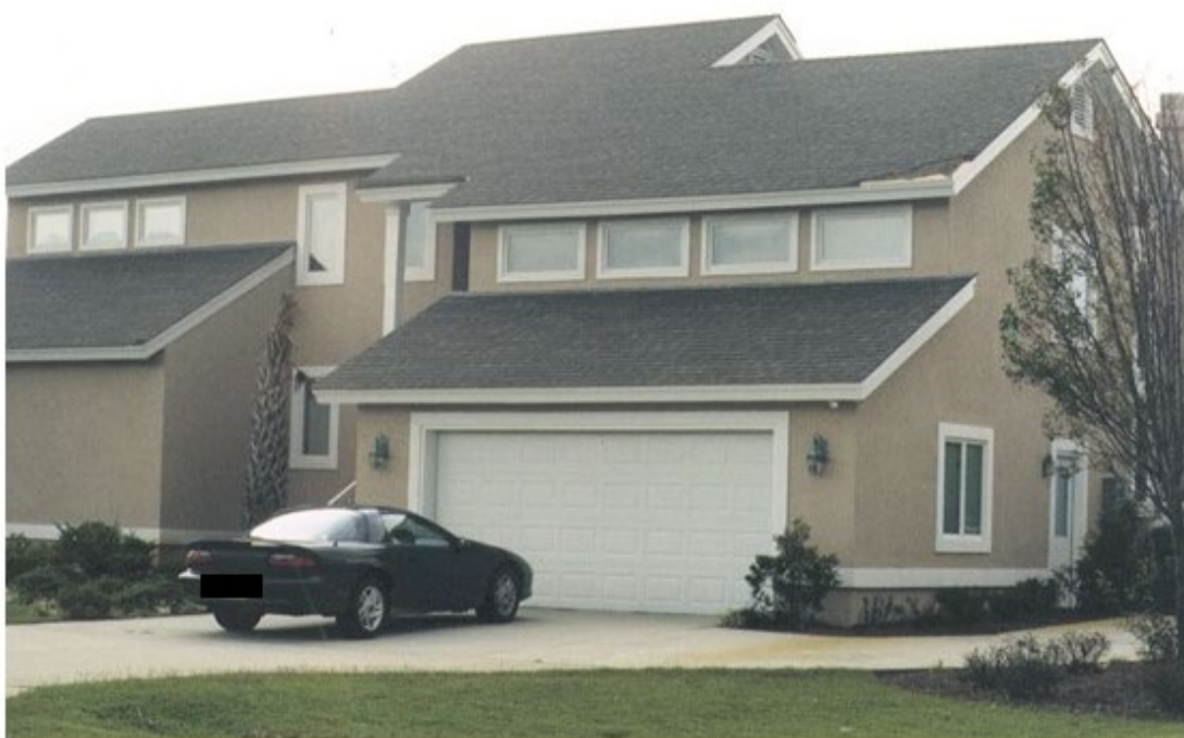
A) <2% Roof Cover
