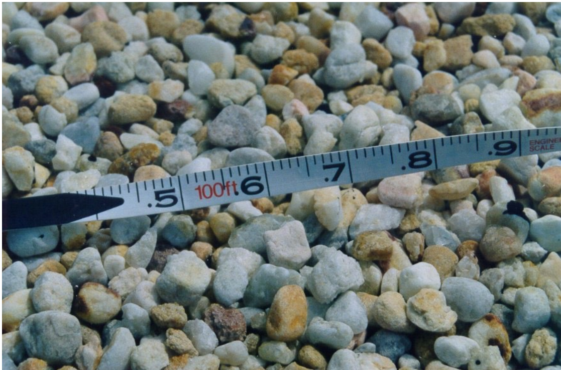
Figure 5-56 Roof Gravel on the Upstream Building
