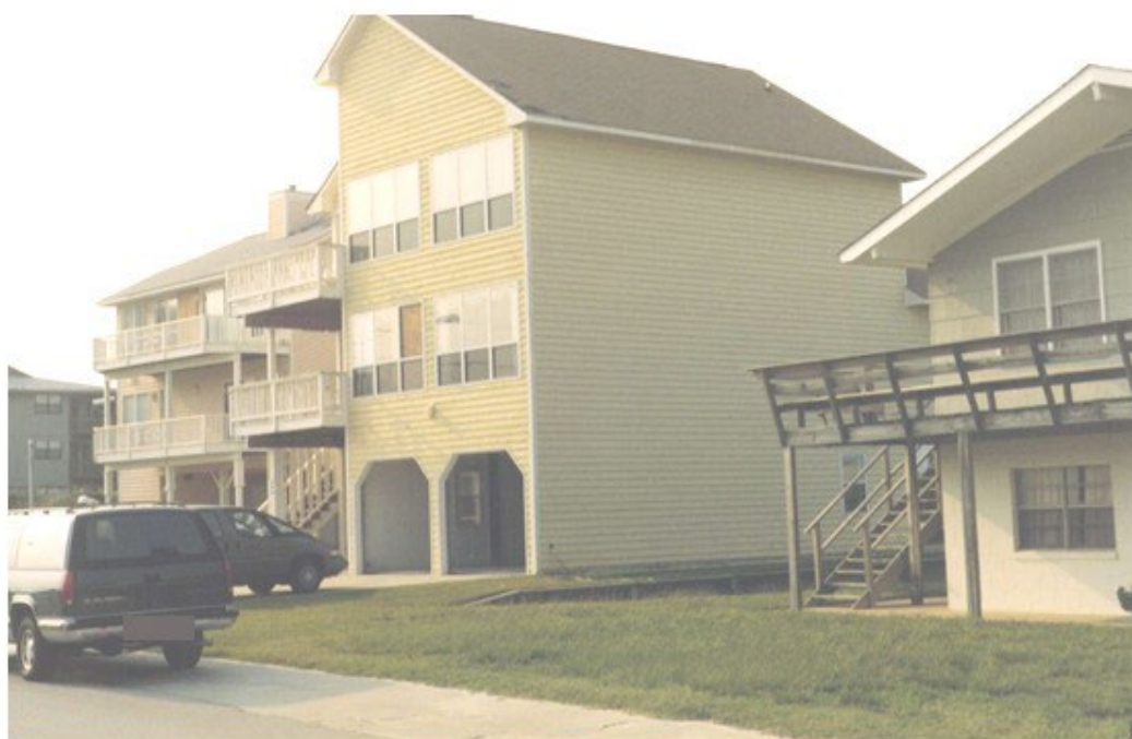
D) One Broken Window
