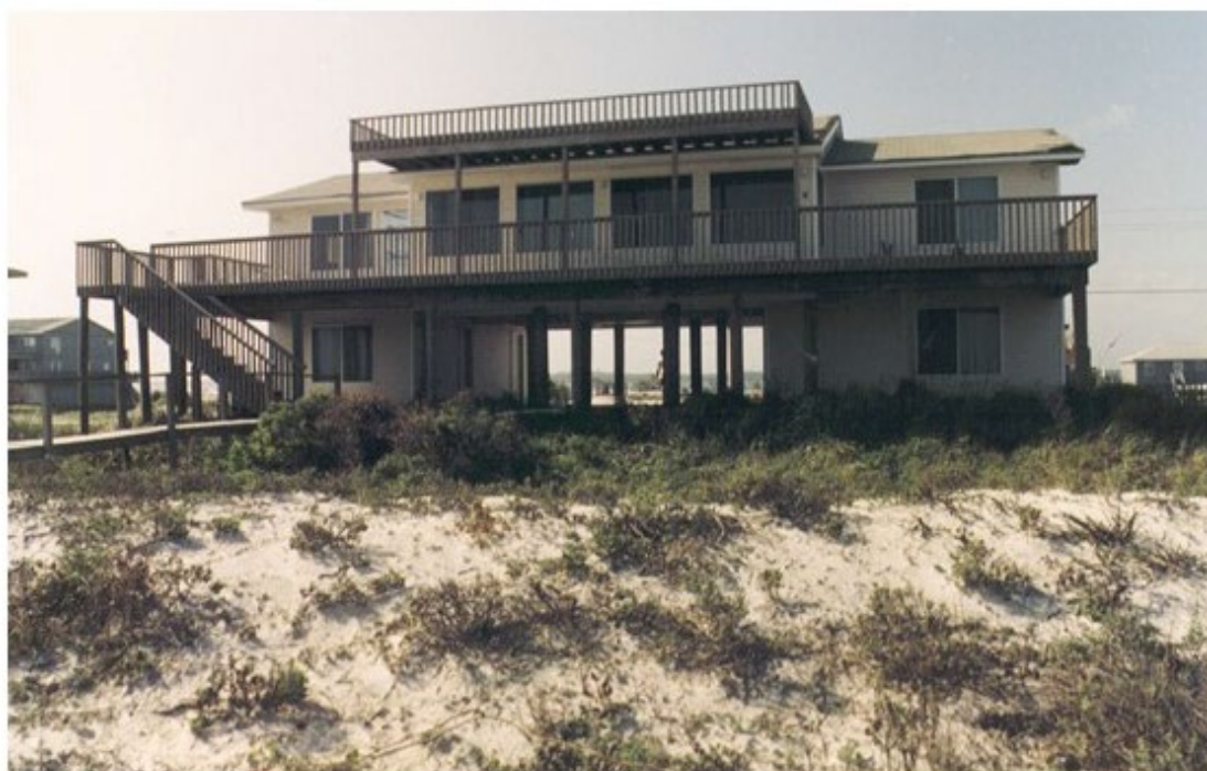
B) <2% Roof Cover
