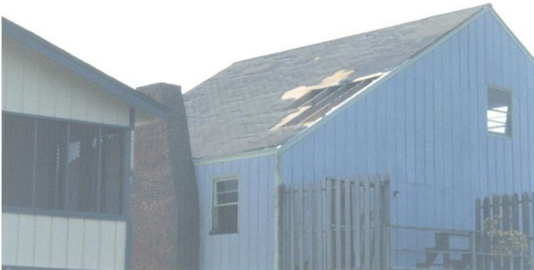
B) At least One Failed Sheathing but Less than Three Failed Pieces of Roof Sheathing
