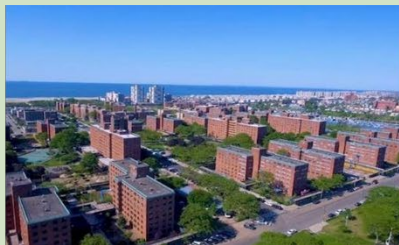
An aerial image of the Ocean Bay Housing Development in New York City.
