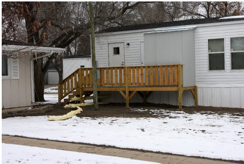
Figure 5: A FEMA manufactured home placed on private property. Photo: Bob Kaufmann/FEMA
