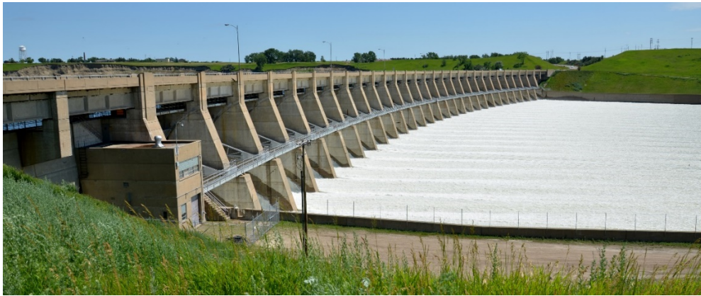
Figure 1: The Garrison Dam Emergency Spillway was opened for the first time ever. Peak flow through the Dam was 180,000 cubic feet per second. Photo: Bob Kaufmann/FEMA
