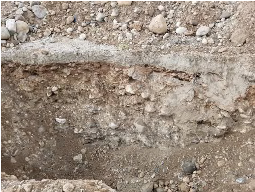
Photo 2. View of conditions encountered in Exploratory Pit EP-1.
