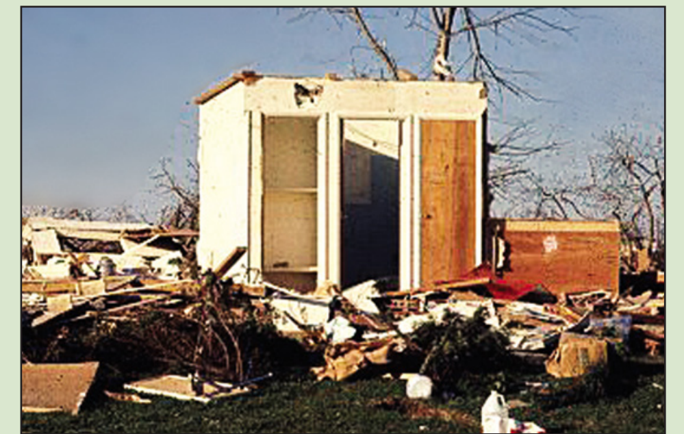
Xenia, OH tornado, 1974. Interior rooms that survived a tornado, such as this one, led to the concept of the above-ground safe room.
