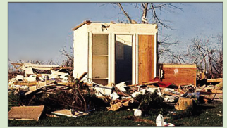
Xenia, OH tornado, 1974. Interior rooms that survived a tornado, such as this one, led to the concept of the above-ground safe room.
