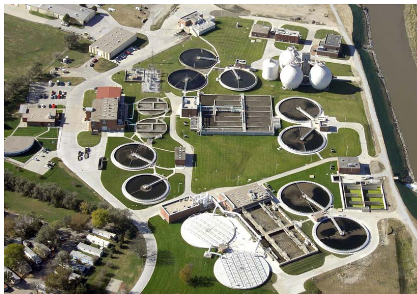
Lincoln, NE's Theresa Street Wastewater Treatment Plant Source: https://www.lincoln.ne.gov/city/ltu/wastewater/treatment.htm
