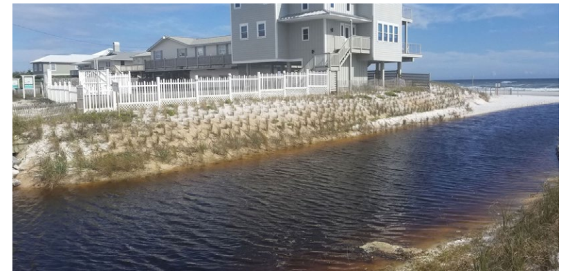
Multiple beach front homes are located at the mouth of the outfall
