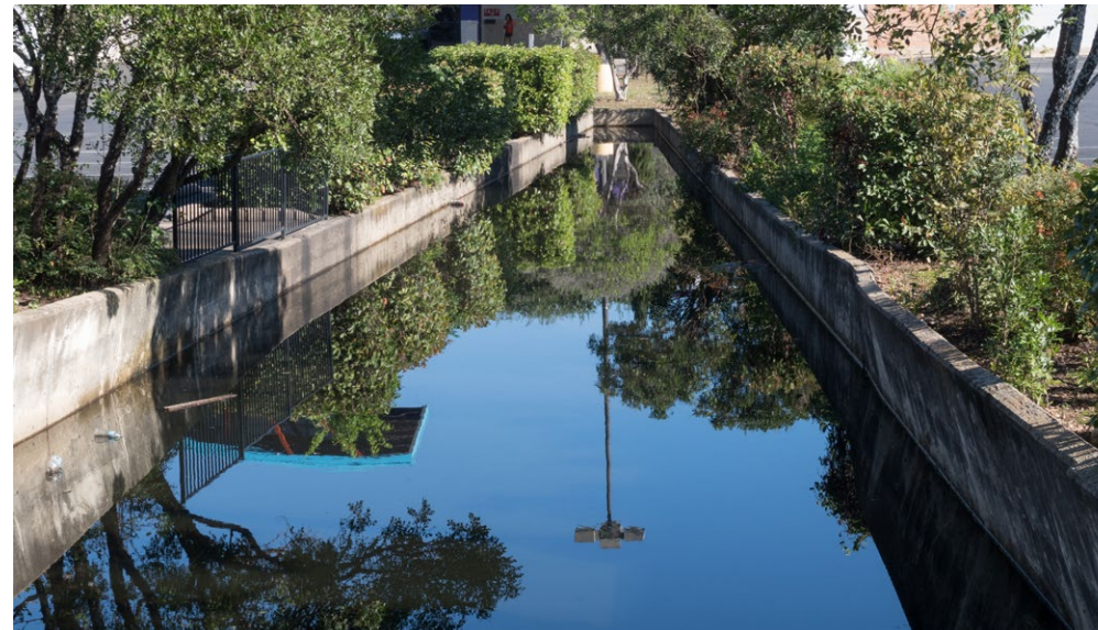
Retention pond used to manage stormwater runoff
