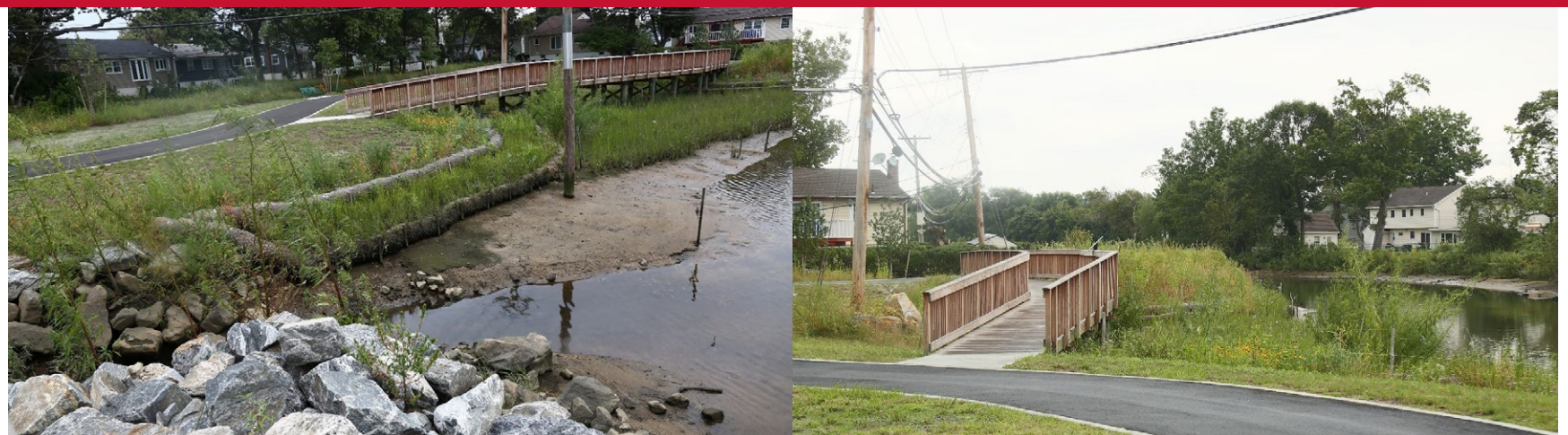
Natural coastal buffer designed to reduce erosion and sedimentation and improve wildlife habitat
