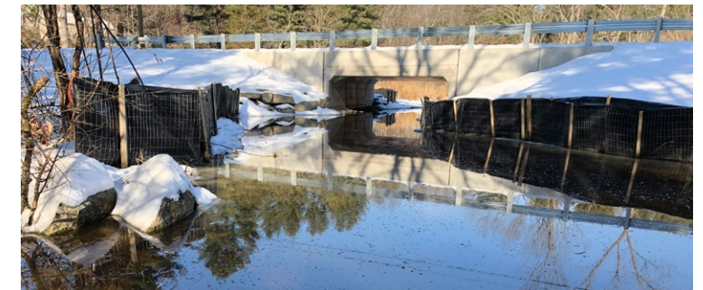
Post-construction high-tide conditions Source: Peter Steckler, use by FEMA is permitted
