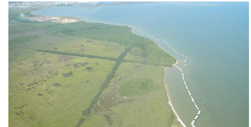
Virginia Point Wetland Restoration Project, aerial view
