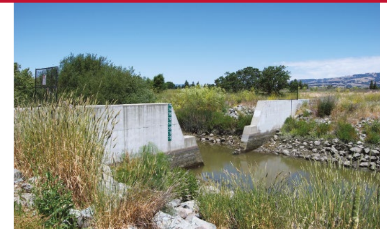
Northern California Flood Control Mitigation
