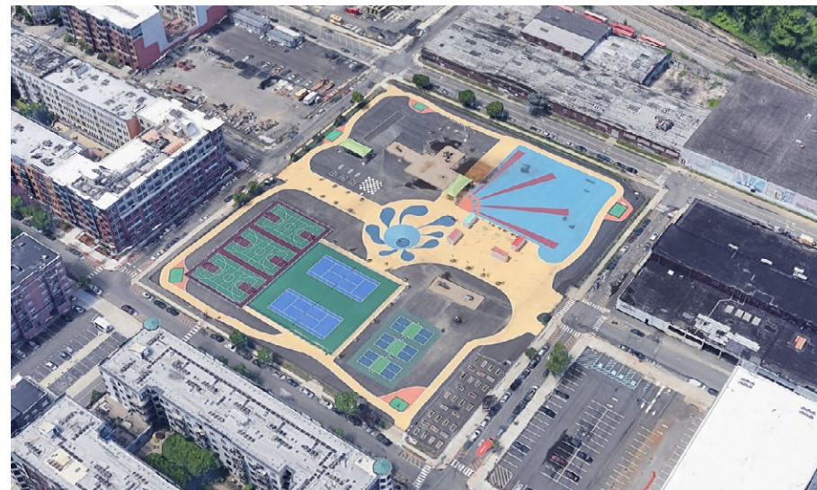
Site of future Northwest Resiliency Park
