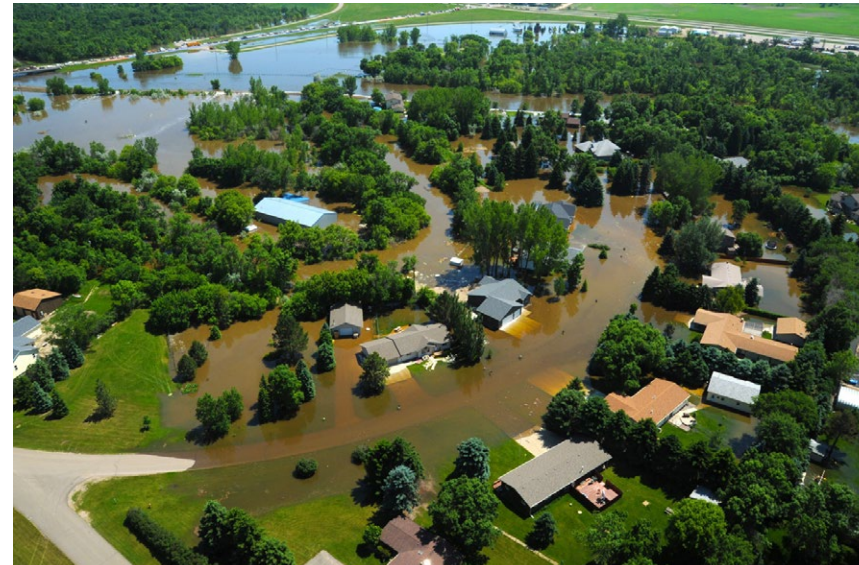
Water floods a neighborhood in Minot, ND, June 23, 2011.
