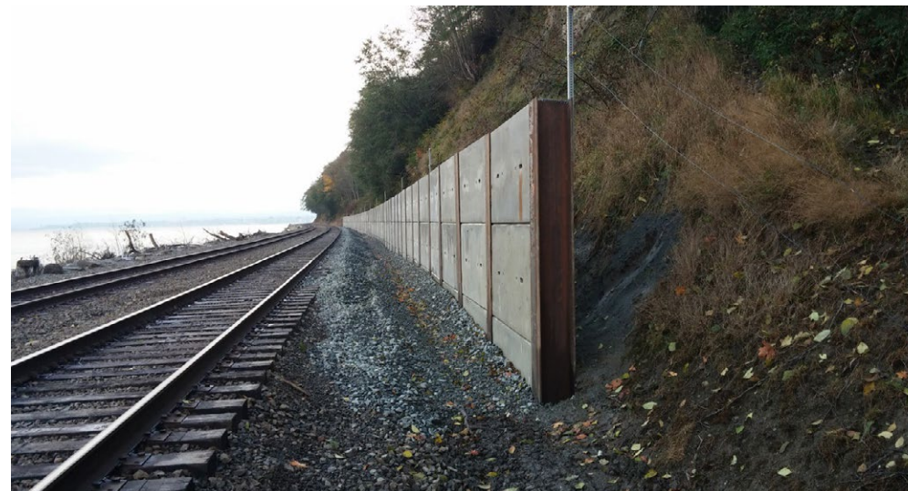
Landslide Mitigation retention wall: The finished metal and concrete landslide retention wall helps keep debris from covering the tracks.
