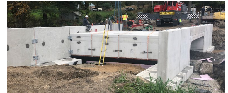
Installation of the last wingwall of the replacement structure Source: Peter Steckler, use by FEMA is permitted
