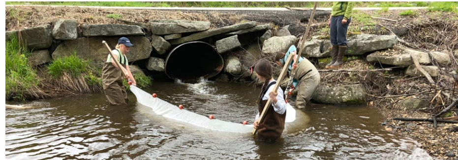
Pre-construction fish monitoring under high tide conditions Source: Peter Steckler, use by FEMA is permitted
