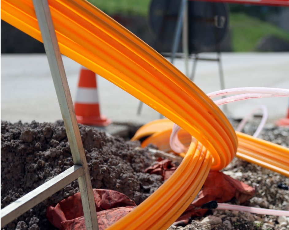
Excavation for the laying of optical fiber Source: Shutterstock
