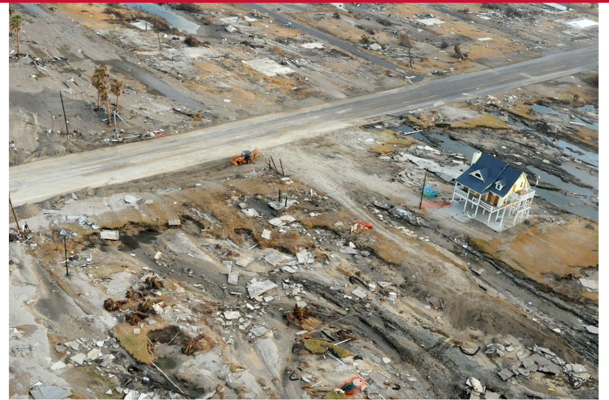
Hurricane destruction surrounding a standing house Source: Jocelyn Augustino/FEMA / Public domain, https://upload.wikimedia.org/wikipedia/commons/5/55/Hurricane_Ike_Gilchrist_damage_edit.jpg
