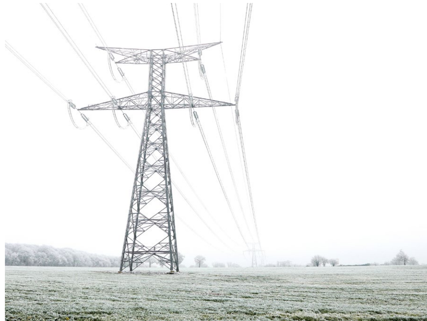
Ice covers electrical sources
