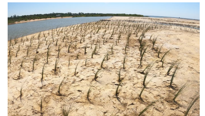
Newly installed black needlerush plugs on edge of the eastern lagoon on Lightning Point Restoration site
