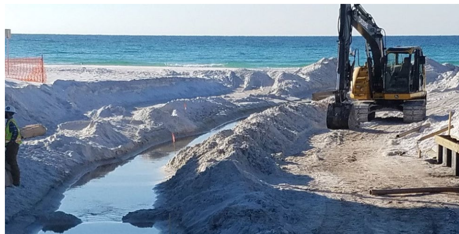
Erosion and sedimentation caused by previous storms and urban growth were straining Oyster Lake's outfall
