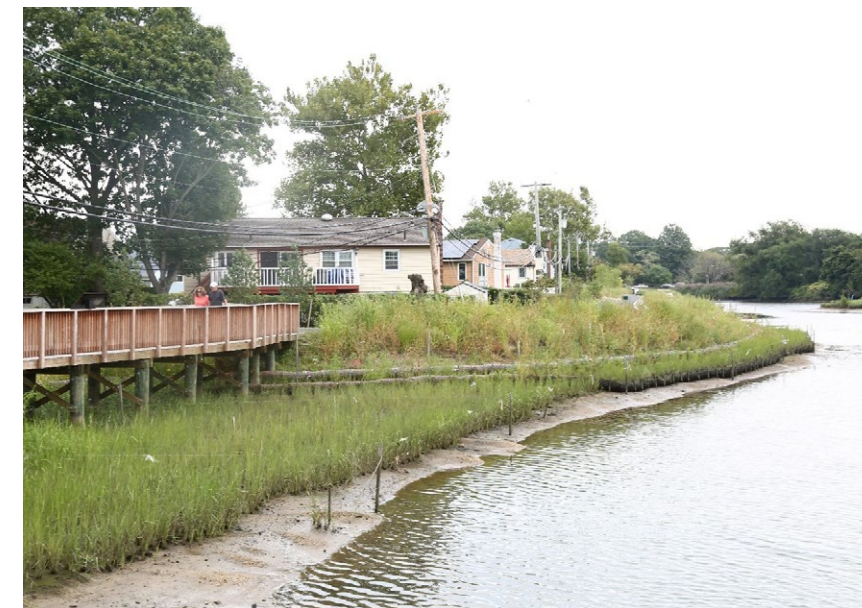
Natural coastal buffer designed to reduce erosion and sedimentation and improve wildlife habitat Source: NYRCR
