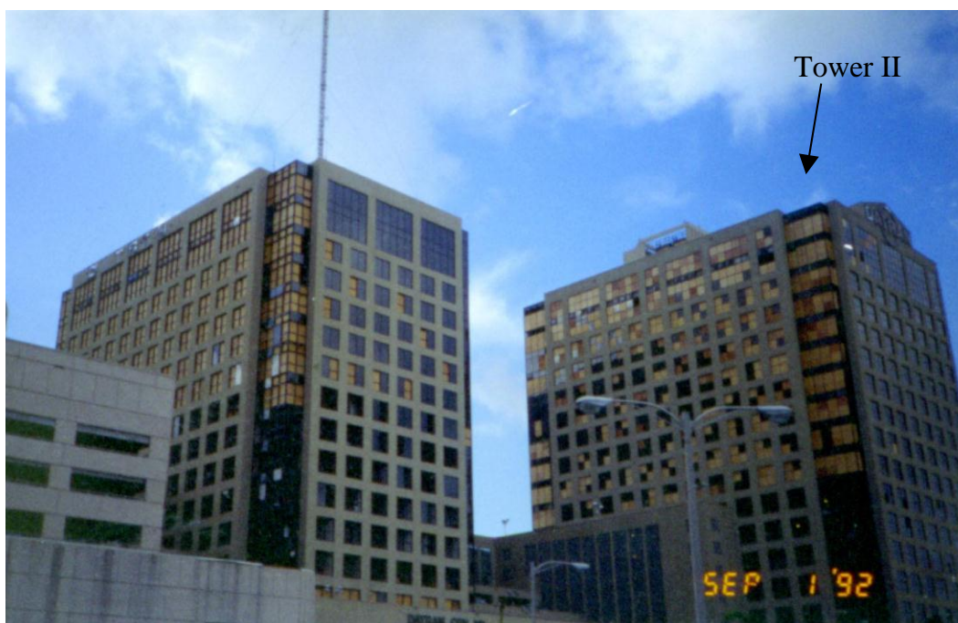
(b) Datran Towers I and II, Plywood Boarding of Broken Windows Complete Except for Lower Floors (Courtesy of TlSmith Consulting).
