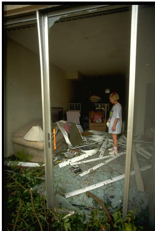
Figure 7.4. Content Losses Due to Fenestration Breach.
