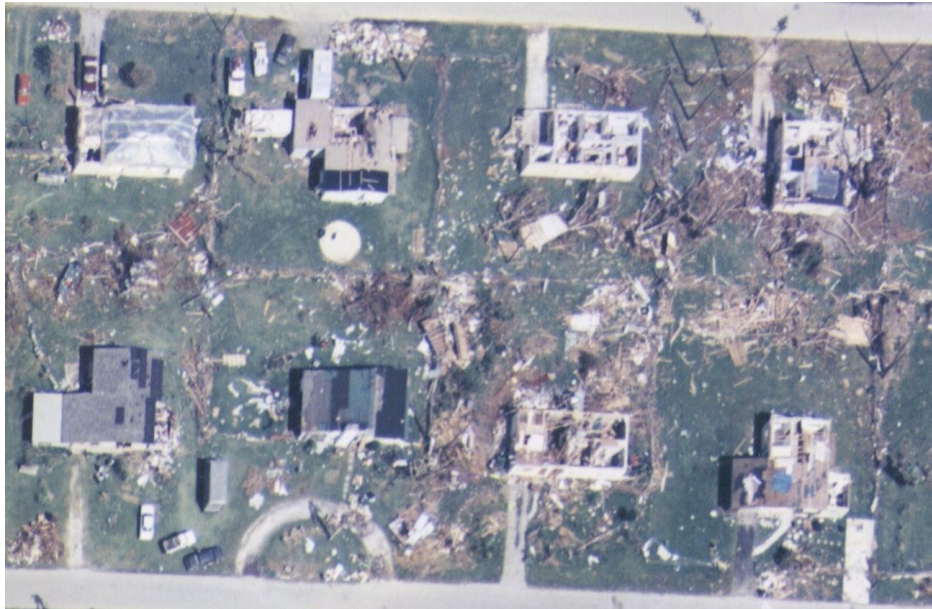
Figure 6-34. Examples of Whole Roof Failures Depicted in Photograph Number 3.
