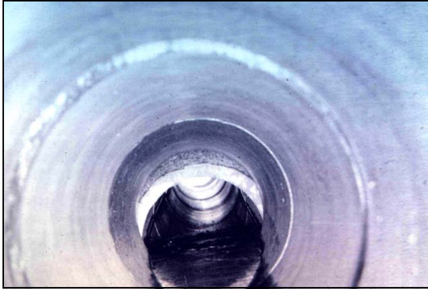
Figure 117. —This conduit was severely damaged after the foundation settled more than 2 feet.
