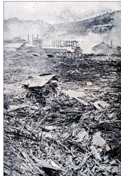
Johnstown, PA, after the dam failure, 1889 (NOAA)
