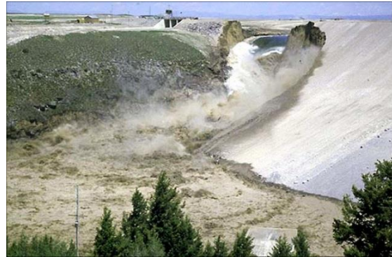
Failure of Teton Dam (Idaho) from seepage (1976)
