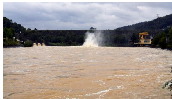
Example of a dam failure
