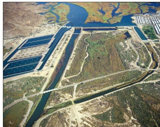
Example of a diversion dam (Imperial Diversion Dam, California/Arizona border) (Bureau of Reclamation)
