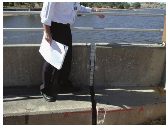
Concrete deterioration
