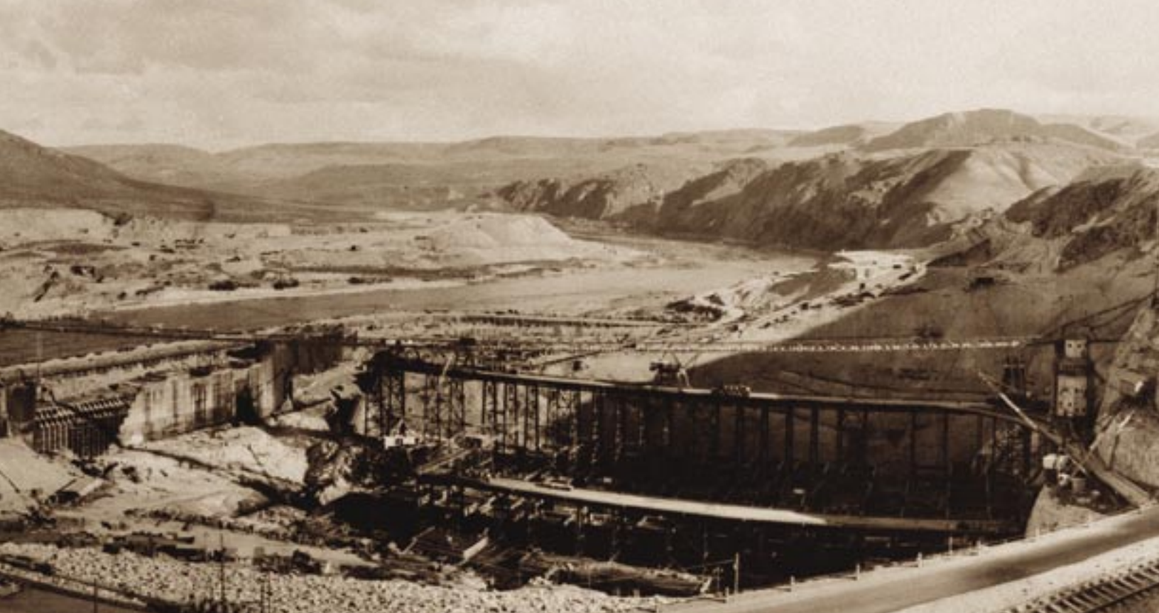
Grand Coulee Dam, Washington. 1936
