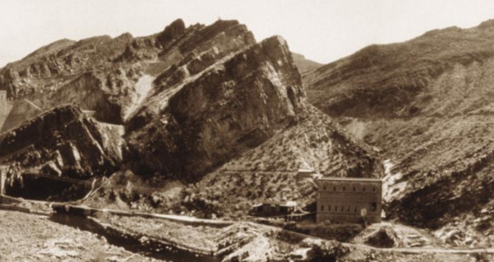
Roosevelt Dam and Power House, Arizona. 1913
