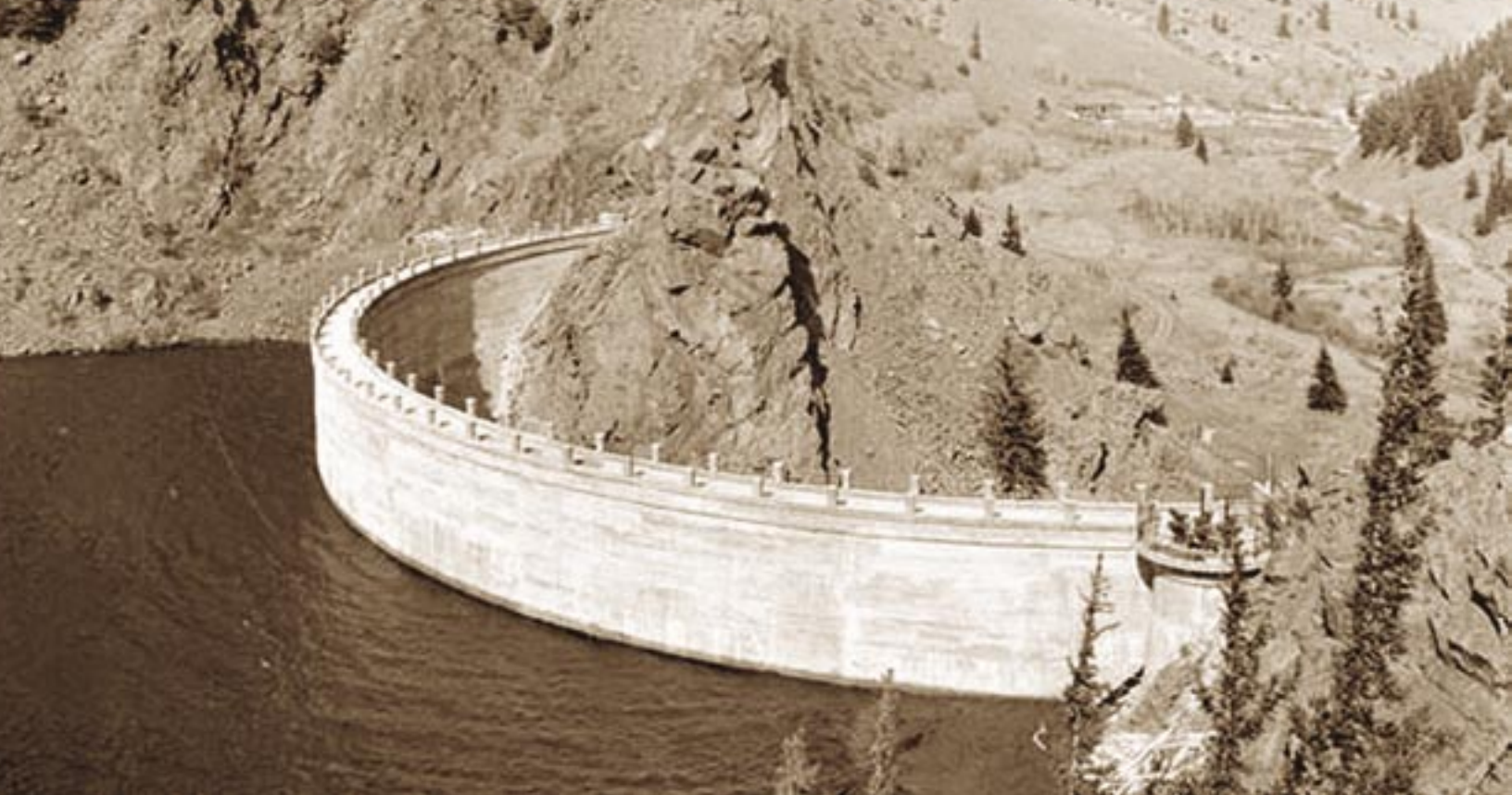
Eaglenest Dam, New Mexico. 1922
