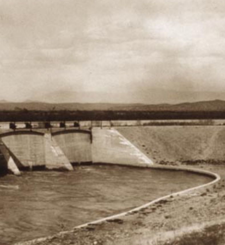
Granite Reef Diversion Dam of the Salt River Project, Arizona. 1913
