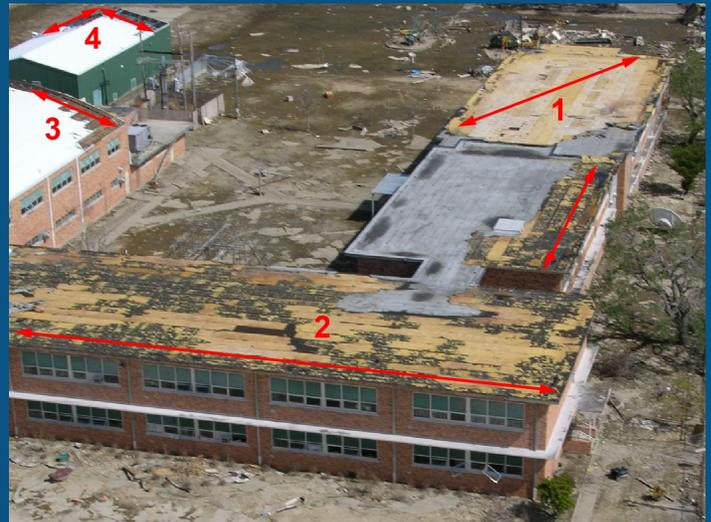
Figure 4. View of damaged school. Four buildings are numbered. Red arrows indicate areas where the roof membrane (Buildings 1-3) or metal roof panels (Building 4) blew off.
