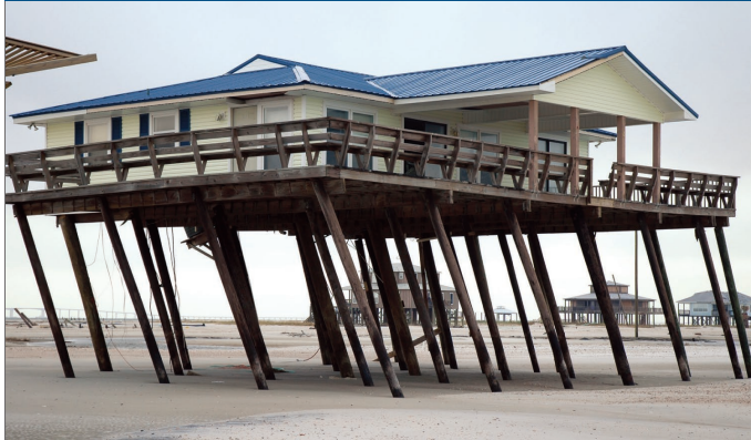
Successful Pile Foundation
