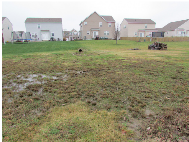
Figure 5.6. Wood debris stored in a stormwater retention area could clog the drainage outlet, threatening the integrity of the retention area berm and causing more significant flooding (Chad Berginnis)
