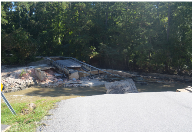
Figure 5.2. Cary Lake dam failure (when this dam breached, 15 properties lost roadway access to the properties) (Maria Cox Lamm)
