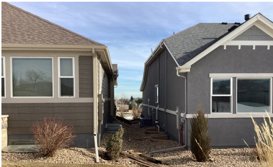
Figure 22. Example of limited separation distances between residential buildings in Coal Creek Crossing in Superior Colorado.
