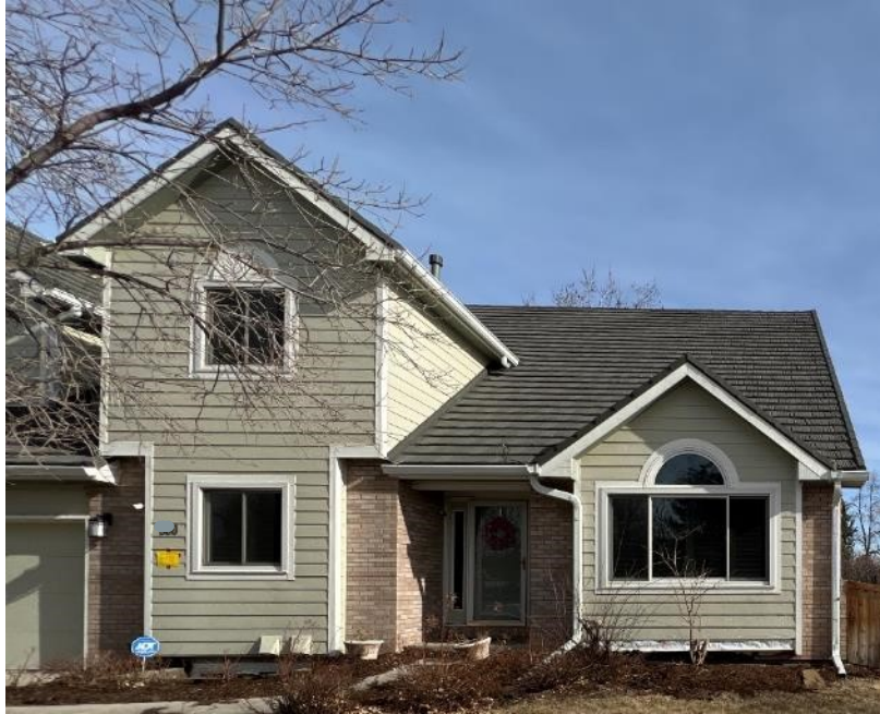
Figure 26. Typical roof system in the Boulder, Colorado area. Roofs tend to have multiple levels, peaks, gables, and joints where debris can accumulate and be ignited by embers.
