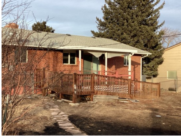
Figure 50. Combustible decking directly attached to a single-family residence in Old Town in Superior, Colorado.
