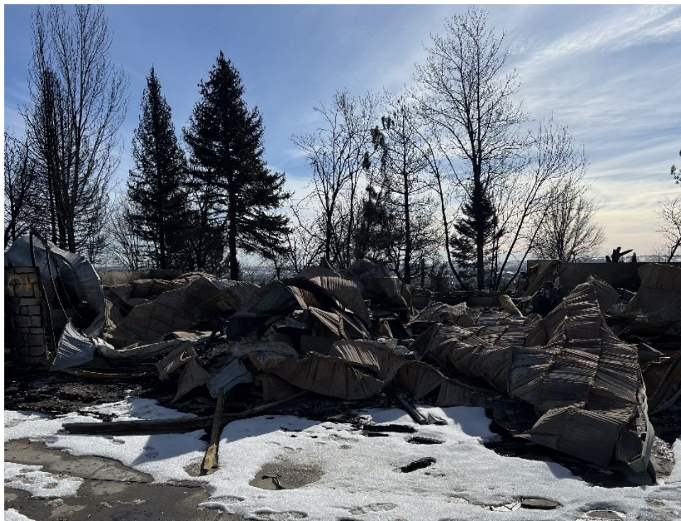
Figure 25. Remains of a residential structure with a metal shingle roof system.
