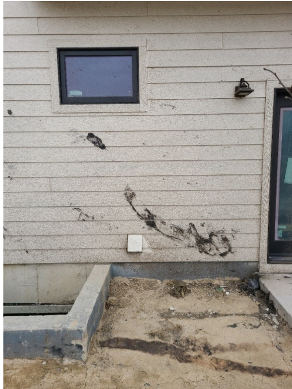
Figure 40. Some homes with fiber cement siding showed evidence of ember impacts to the exterior facade but did not burn. In this case, the base of the wall system had little to no combustible fuels providing the embers a fuel bed for ignition.
