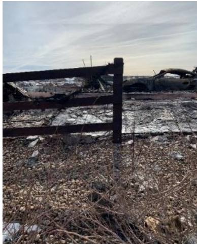
Figure 54. Fences behind communities may have acted as wicks, drawing fire to the neighborhoods.
