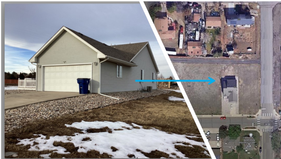
Figure 20. Example of a single-family home in Old Town in Superior, Colorado where ample defensible space and structure-to-structure separation likely contributed to its survival when numerous structures in the neighborhood were completely destroyed.
