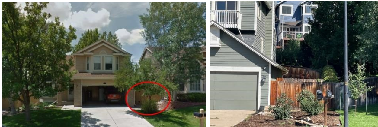
Figure 53. Additional examples of combustible fencing attached directly to single-family residences in Louisville, Colorado.
