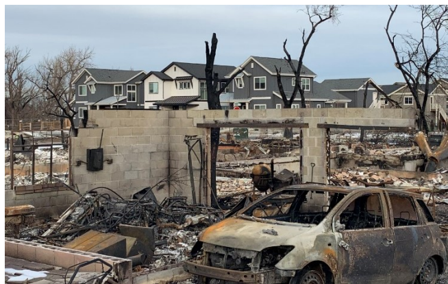
Figure 39. Concrete block and brick around garages often remained partially or fully standing.
