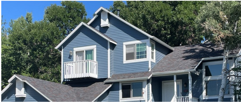
Figure 30. Example of an observed complex roof design.
