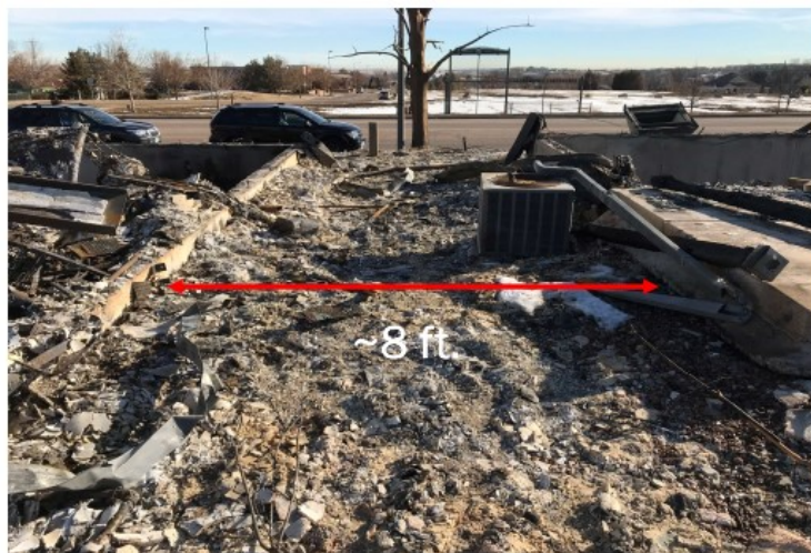
Figure 23. Additional example of limited separation distances between residential buildings in the Sagamore neighborhood in Superior, Colorado.
