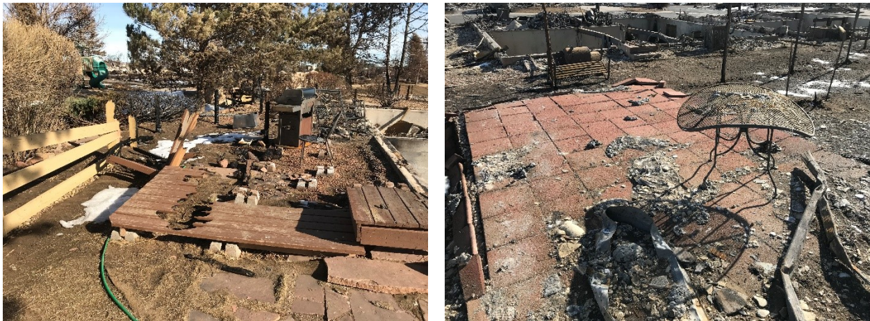
Figure 48. Patios often contained furniture and grill propane tanks which are known to contribute to fire spread.
