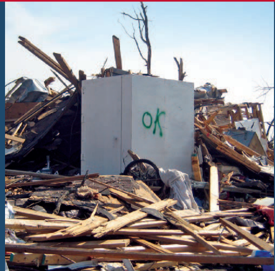
Above-ground residential safe room that was in the garage of a home hit by an EF5 tornado in Joplin, MO (2011)
